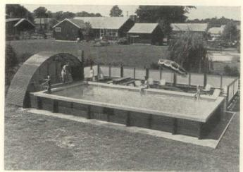
Cabana pool can be used on poor terrain, needs only diving-end excavation. Redwood walls support pool 3' above ground. Vinyl bottom liner rests on composition floor. Fiberglass side walls admit underwater light. Walk around pool is concrete, 3' wide. Cabana 8'x16' is at diving end. Filter and heater go under cabana. Ladder is hinged. Vacuum cleaning system is built in. 16'x32' pool can be built for less than \$1,000 materials cost.
