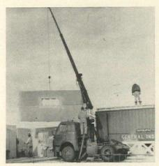
Versa-Lift crane is specially designed for handling prefab components, is mounted on 1½-ton truck or on prefabber's trailer rig as shown here. Boom extends from 8' to 30', will lift 7000 lb at 8', 650 lb at 30', can swing full 360°. Hydraulic pump is driven through a power take-off. Remote controls are available.
