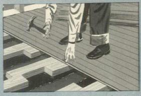
Screeds laid in mastic provide nailing surface for installing Strip Oak Floors in homes built on concrete slabs. Write National Oak Flooring Manufacturers' Association for free installation manual.
