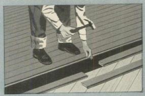
Simplest of all floors to install, Oak is nailed to subfloor in wood joist construction. Modern Strip Oak Floors are precision manufactured in a variety of sizes and grades to suit any building requirement.
