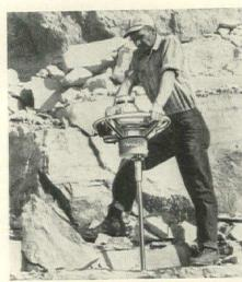
Winkie core drill weighs 45 lb, is 19" high, 21" wide. A 2-cycle 5½-hp gasoline engine provides bit speeds of 2000 rpm. In shallow drilling the unit can recover 8" cores, can recover 15/16" cores down to 200'. Standard core lengths run to 18". Winkie can also drill holes in masonry. Price: \$900.
