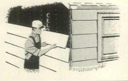
HARDBOARD SIDINGS. Beautiful, durable, easy to paint. Channel-Lap\* applies with aluminum channels; factory primed; invisibly fastened; self-ventilating. Verti-Groove\* offers vertical plank effect. Texbord\* striated surface panels or shingles.
