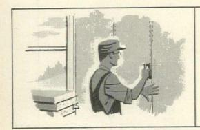
MINERAL WOOL BLANKETS. Preferred ceiling and wall insulation. Spun-Process manufactured for lighter weight, extra resiliency. Built-in vapor barrier. Reflective and regular types. Full, medium and utility thicknesses.
