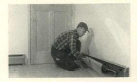
Kumpf shows how the cover of the Art Comfortline Baseboard is extended the length of the wall, even though less radiation than this is needed.
