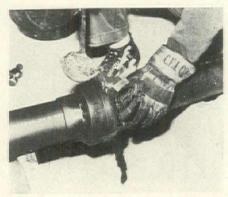
Carlon pipe fitting allows hot-lead joining of plastic and cast-iron sewer pipe. Fitting is solvent welded to plastic pipe. Bell end is packed with oakum and wrapped with asbestos rope before lead is poured around the metal pipe to form permanent connection.
