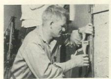
Pop-up rivets fasten lightweight metals, plastics, or sheet materials in gutter systems, wall panels, ductwork, etc, in blind or limited access spots. The rivet is a heavy hollow shank which is expanded by a mandrel when it is pulled into or through it, making either a solid seal or a through hole. Rivets cost about 1¢ a piece but installation is very fast and labor savings high.
