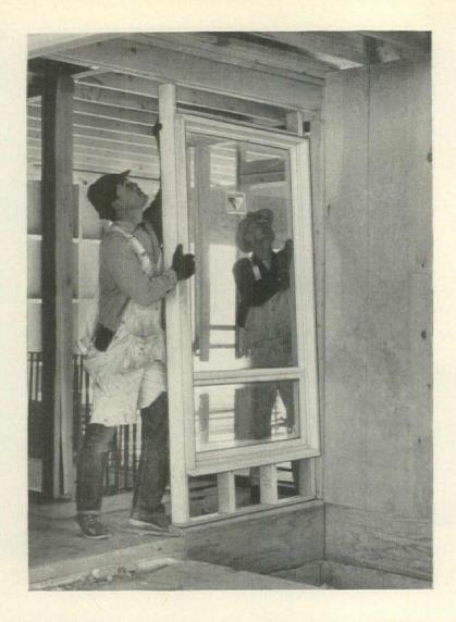
Tilt up wall construction and the use of the new, modular Andersen Strutwalls were big factors in bringing the huge job in on time.
