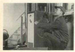
Contractor W. J. Kumpf hooks up the National-U.S. "11-B" Series cast iron boiler in three-level house built by Edward M. Ryan in Pittsburgh.
