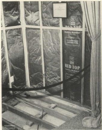
CORNER CUTAWAY shows wall insulation and unorthodox floor construction—wood floor is laid on sleepers over slab foundation.
