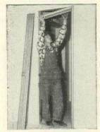
Snap hinge jamb over stud and wallboard. Snap header into opening with hinge jamb. Install strike jamb same as hinge jamb.
