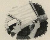
Fold ends of blanket and fasten to sill plates on either side, sealing the insulation. Fold the flanges over the face of the studs to close the edges. Final seal is made when gypsum board is applied.
