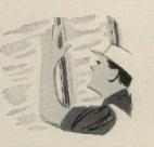
Fold flanges over the face of the studs to close the edges. Final seal is made when gypsum board is applied.
