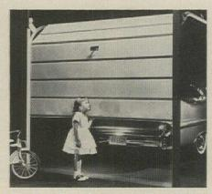
Steel roller door is built so folding sections will push your hand or fingers out of the way when door is closing. Panels are galvanized, bonderized, and prime painted on both sides, are held in alignment by full width hinges. Nylon rollers are locked in a tapered track. Bottom weatherstrip is vinyl. Five-year warranty. Price \$69 for single-car door.
