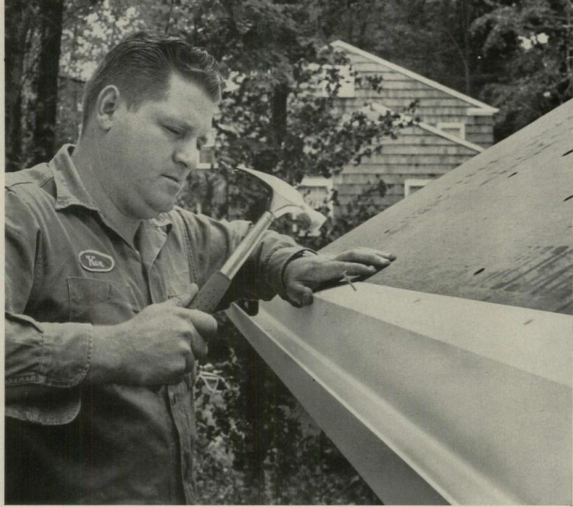
EXCLUSIVE FLASHING FEATURE! No other gutter has its own flashing that fits right under the first row of shingles. Eliminates the need for a drip edge. Saves time, money and extra labor!
