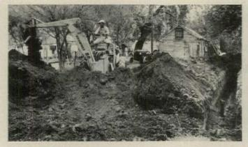
**Shawnee 88 backhoe** is a new high-speed digging tool. Two single-acting cylinders give uninterrupted 188° swing, keep chain under tension to prevent slop and compensate for wear. Bucket cylinder is hidden in the 88's bucket boom so it will not be damaged and cause job delays.
