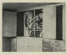
**3.** Where the attic space is limited, fan may be installed in basement or sidewall for efficient whole-house ventilation.
