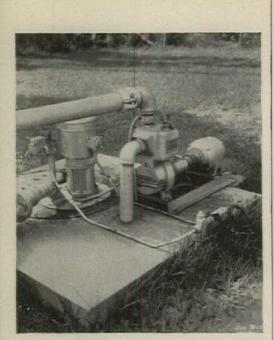
In Jacksonville, Fla., a 3-inch Gorman-Rupp Sewage Pump replaced a vertical pump after 21/2 years in service.
