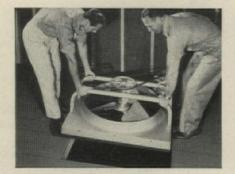
1. In normal installation, R&M-Hunter Fan (Package Type) is placed on attic floor with automatic shutter in hallway ceiling.
