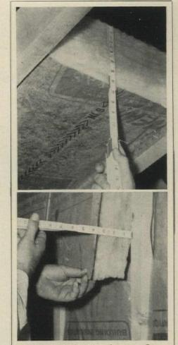
**REQUIRED INSULATION** in every Owens-Corning test house was: 1) 3" foil-wrapped batts or 6" bulk insulation over ceilings (photo top of page); 2) 3" batts in outside walls (photo above); 3) 2" to 3" for floors—like the 2" perimeter insulation for crawl-space walls shown below.
