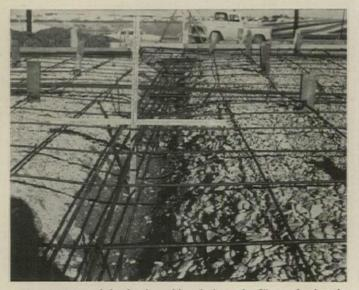
**BEFORE POUR**, reinforcing is positioned above the 5" gravel subgrade by wooden blocking which is removed as concrete is being puddled.
