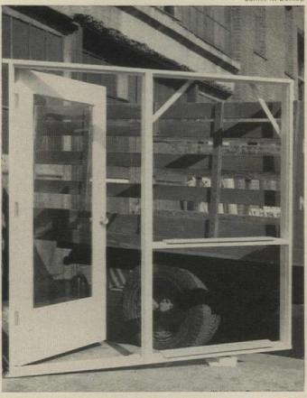
**DOOR-AND-WINDOW COMPONENT** for Bennett houses was built to architect's specifications by Lamar & Wallace, local millwork company.
