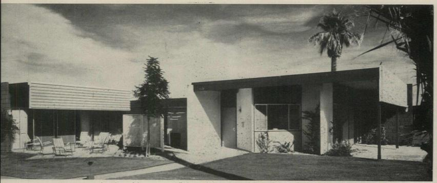
EACH BUILDING is made up of three apartments. Earlap overhangs, a trademark of Architects Palmer & Krisel, fend off rays of low sun.
