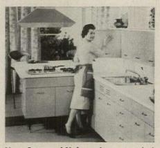
New Geneva kitchens have an etched crackle finish designed to give a look of warmth to steel cabinets. The new finish is claimed to be chip, scratch, and mar proof. It comes in a wide variety of colors. Sound-deadening material in door and drawer fronts, nylon drawer rollers, and plastisol-coated shelves help make these kitchens especially quiet.
