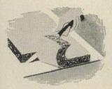
Measure length of material. Allow 3 or 4 in. for end flanges. Cut with insulation laid on a flat surface. Foil flanges can be formed by cutting away fibrous material.
