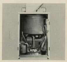
**Timed bleach injection** is a new feature in 1959 Maytag washers. A measured amount of bleach is poured into an opening at the top of the washer, runs down a tube into a dilution reservoir which fills with water as the tub fills. As the washing begins the diluted bleach is drawn into the inner tub at a controlled rate to insure good but safe bleaching. Maytag Co, Newton, Iowa.
