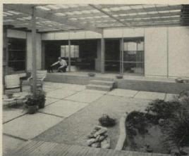
**COVERED PATIO** in Ryan house is sheltered beneath reinforced plastic roof supported by rafters.
