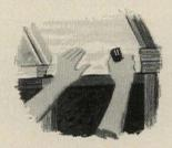
Install ceiling insulation using same technique, except that air space is  $1\frac{1}{2}$  in. or more depending on the width of the flange. The greater the air space in the ceiling, the greater the insulation effectiveness. In walls, this space must not exceed  $\frac{3}{2}$  in. For ceiling insulation, the sides are normally secured before the ends.
