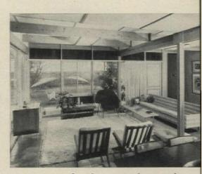
**DOUBLE 2x10's** form beam supporting exposed joists in the living room of a \$21,000 Ryan house.
