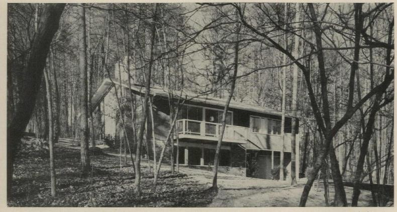
BENNETT'S "OVERLOOK" MODEL was designed for an uphill site. Front entry, left of garage, is sheltered by cantilevered upper level.
