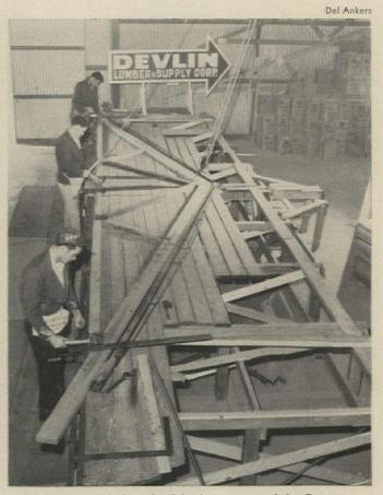
**ROOF TRUSS**, made by a local lumber company, helps Bennett meet 61-day building schedule although he builds many custom-type houses.
