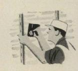
Follow same procedure for wall insulation, except that air space between gypsum board and foil vapor barrier should not be more than  $\frac{1}{2}$  in. Top and bottom of blanket are usually secured first.
