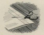
Measure length of material required, allowing 3 or 4 in. for end flange. Cut or tear.
