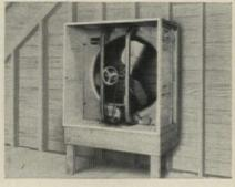
**2.** In gabled homes, where attic is airtight, the "A" Type Fan can be mounted as shown to discharge directly to outside.
