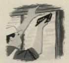
Press blanket firmly into stud space and fasten to the sill plate with staples to form a <sup>3</sup>/<sub>4</sub>-in. air space between the gypsum board and vapor barrier.
