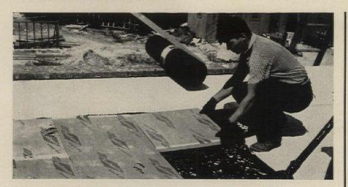
Dow roof insulation, called Roofmate, is Styrofoam plank wrapped in laminated kraft paper. Boards are 2'x4', and may be 1", 11/4", 15/8", or 2" thick. Light weight, high compressive strength,
