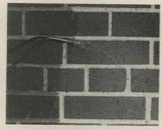
Silicone water repellent from Dow is claimed to give five-year service. Dow Corning 770 can be diluted with plain mineral spirits, is as clear as water, is effective on mortar, brick, concrete, or other masonry. The new repellent is shipped as 33% solids, is available now at competitive prices in any quantity. Dow Corning, Midland, Mich.
