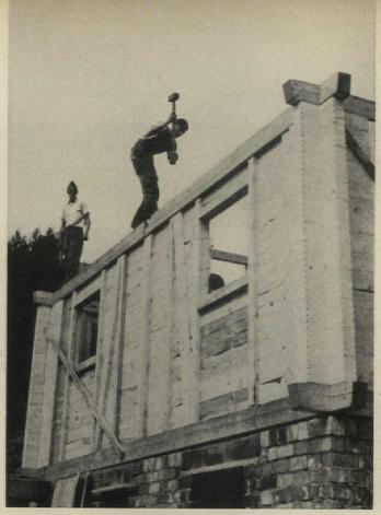
**WALL PLATE** is interlocked with partition (seen through window), then fastened with dowels, shown being hammered in. Partitions are plastered. This stage marks end of second day of construction.
