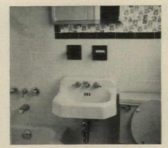
BATHROOM tiles are glued to Masonite skin; hardware and pipes are cut into panels, through to plumbing space behind.
