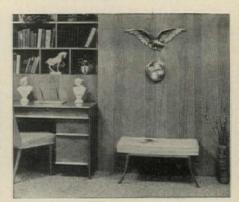
**Varied grain paneling** is actually  $\frac{1}{4}''$  plywood in standard  $\frac{4'x7'}{4}$ ,  $\frac{4'x10'}{x8'}$ ,  $\frac{4'x10'}{x10'}$  sizes. Choice wood grains are photographed and transferred to the plywood sheet in nine-plank patterns, with or without V-grooves. Various finishes are available (above, colonial oak). The paneling is guaranteed against fading, structural defect, or delamination for the life of the installation.
