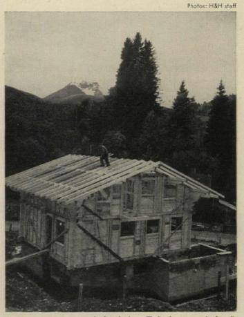
**ROOF FRAMING** goes on in fourth day. Chalet is now ready for tile roof and final trim and finish. This chalet has a concrete basement for utilities. The finished house has 1,800 sq ft, cost \$20,000.
