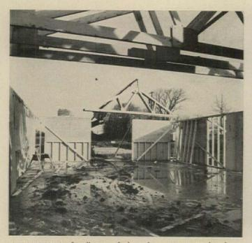
**OPEN SECTION** of wall, rear of photo, lets tractor move into house with load of trusses. Tractor sets trusses on plate where carpenters quickly fix them in position. Framed wall section, leaning against wall at right, will be used later to fill the opening.
