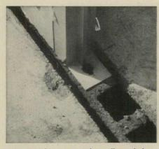
COLUMNS between exterior wall panels have welded base plate held by anchor bolts to block foundation. Panels sit between columns, are not tied to foundation (see opposite).
