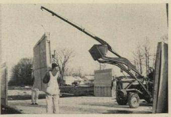
**HIGH-LIFT** boom—now on slab—reaches into trailer to snake off heavy wall panels and move each to its place. Remainder of load seen on trailer includes plywood sheets stacked under inverted trusses at front of trailer, precut studs near tailgate, and trim material between trusses and panels at right.
