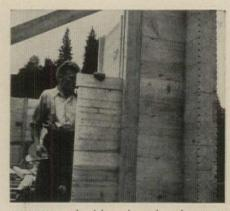
**SHEATHING** is driven into slots in corner construction. Corners go up first. Photo shows work in afternoon of first day.
