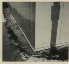
EXTERIOR WALL has special corner panels fabricated in 'L' shape. Finish is a baked alkyd enamel on aluminum skin. Drip cap extrusion covers sill-line joint.
