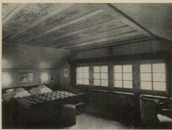
**Decorated ceiling** is over bedroom in chalet Bärglimatt (Gstaad), built in 1647. Battens are  $\frac{1}{2}$  meter (approx 20") oc, were milled from 2"x4" stock. The traditional flower and foliage pattern is painted on the panels in soft pastel tones. Bracket at right extends up to ridge, and out to deep gable overhang. Note traditional hardware on windows.
