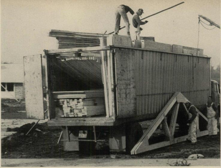
TRAILER-LOAD of components, plywood, and precut studs for a house is backed into "L" of slab to get materials close to point of use.
