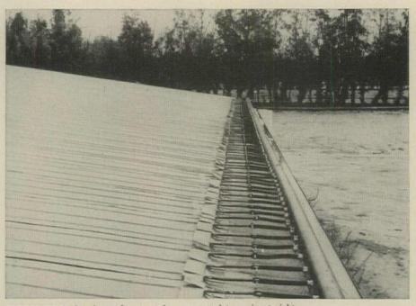
COPPER ROOF has integral water tubes connected to main at right.
