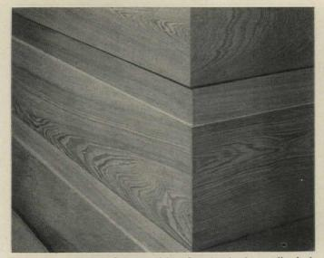
"MITERED CORNERS give you a tighter fit and make the paneling look as though it is all out of the same wood mass. Each cut takes a lot of fitting. It took four cuts on the machine to get this paneling."
