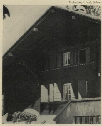
**Gable overhang** on Chalet Bärglimatt is 8' deep. It is supported by huge bracket spanned by purlins. This chalet is now roofed with shingles, but originally had a slate roof. Rocks are often placed on chalet roofs to hold them down in strong winds. The  $25^{\circ}$  roof pitch keeps snow on the roof for insulation (chalets were not well heated until recently). The deep gable overhang protects the end walls, with all their joints, from the weather.
