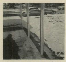
**COLUMNS** supporting carport overhang are the same as columns used at every panel joint in exterior wall and center bearing wall. The hollow members are one-piece extrusions.
