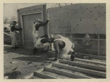
**ON SITE**, framing for solid wall is made from pre-cut studs, as shopbuilt section (at rear) is fitted into place.
