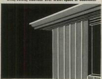
Gutter, Fascia, Board and Batten Siding
