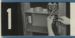
Rough-in box fits 16" O. C. joists and is attached by the adjustable mounting flange or directly to joists. Remove junction box cover, or for existing work the complete box is removed from inside. Rough wiring connections are all that is necessary. Slip duct on removable duct sleeve. Flanges are pre-set ¾" for standard plaster thickness.
