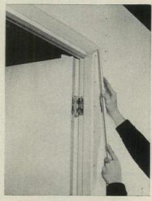
A slip jamb prehung door fits the balsa core panel openings. Plywood spreaders (photo far left) and shims between door edge and jamb hold the door to its jambs-squarely, tightly, and with the right clearance—until the unit is nailed to the panel.
