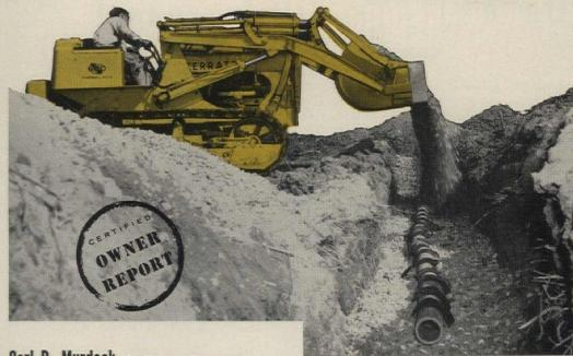
Carl D. Murdock, Indianapolis contractor specializing in residential sewer work, has cut the cost of installing septic systems one-third, by teaming a powerful 1-cu. yd. Case<sup>®</sup> TerraTrac<sup>®</sup> Model 600 crawler-loader, with a versatile Case Model 320 wheel-mounted backhoe-loader combination.
