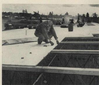
HOW YOU USE PLYCLIPS is shown in this installation of a plywood roof deck on beams 4' o.c. on a new supermarket, a DFPA's test job.
