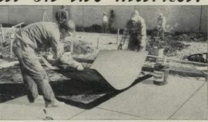
COMPARE the strength..."PM" maintains its permeance rating even after being subjected to the pouring of aggregate, trundling of wheel-barrows and installation foot traffic. Resists rupturing and tearing. How many other materials will perform like this? COMPARE the ease and speed of providing a permanent installation..."PM" may be laid directly over the tamped grade or fill. Ideal for all types of construction; basement, crawl-space and slab-on-grade.
