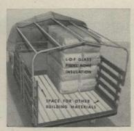
2. Costs less to handle. Compressed rolls take less than half the space of other types of insulation.
