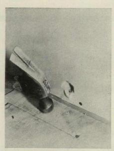
PANELS ARE NAILED to sub-floor by toenailing through drywall and shoe. Dent left by hammer is covered by base molding. Panel can't belly because of grid core.
