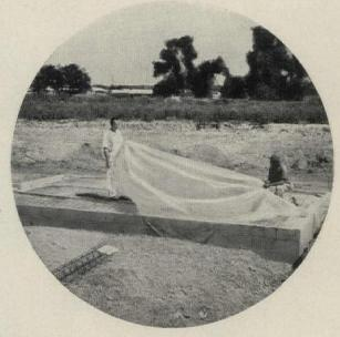
"Olin Polyethylene is the finest moisture barrier we've ever found for use in home slabs," say Zeiger Construction Company, Dayton, Ohio.
