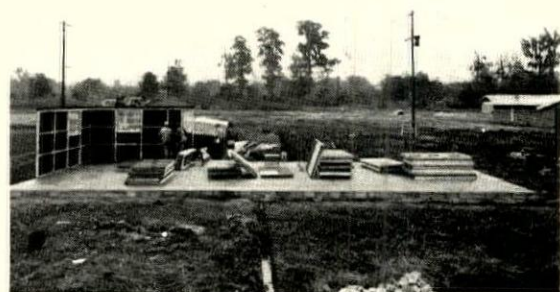
9:10 AM Wall panels are raised on slab.
