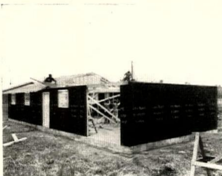
11:30 AM Roof trusses are set on walls.
