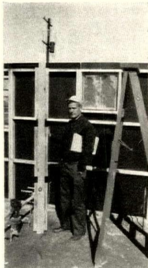
PREBUILT T-POST speeds joining of partitions to wall panels.
