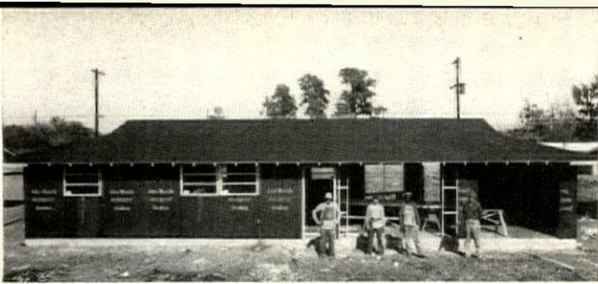
1st day: House is under roof. Then . . .
