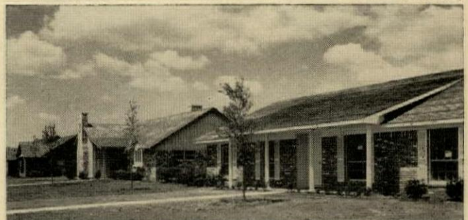
SHARPSTOWN's varied houses were built by over 30 builders.
