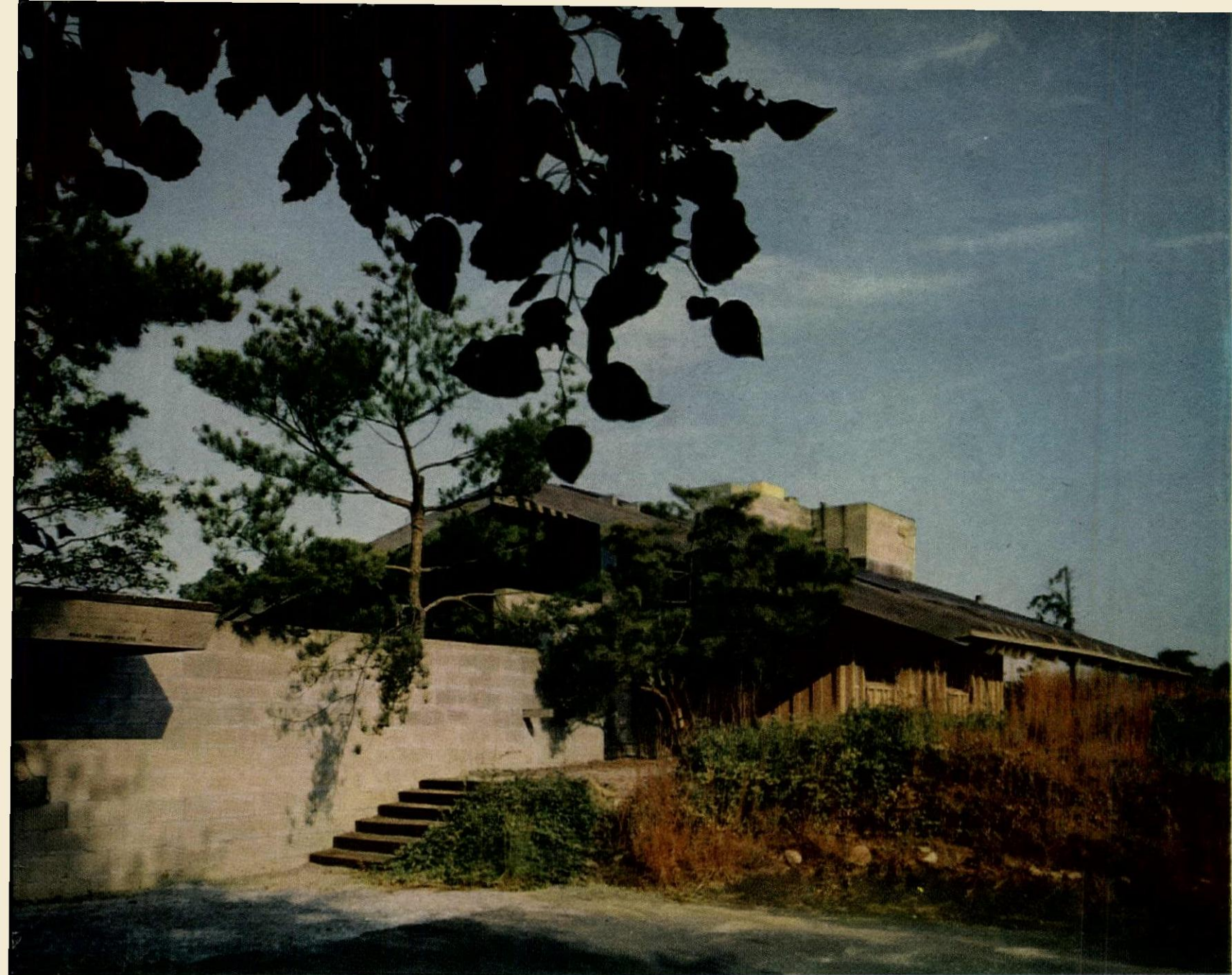
BROAD SLOPING ROOF with low eave line ties country house to its sloping site. Concrete block wall hides living areas from entrance drive.
