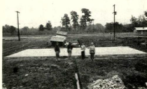
8 AM Men and wall panels arrive at site.
