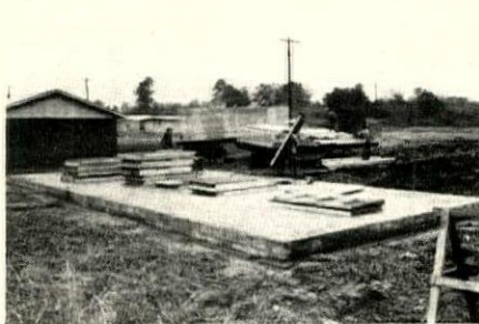
8:20 AM Trailerload of trusses arrives.
