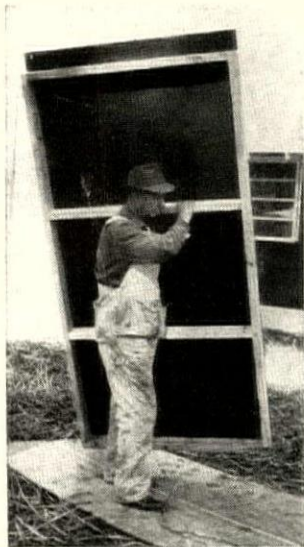
UNUSUAL PANEL has girts to make it easier to man-handle.
