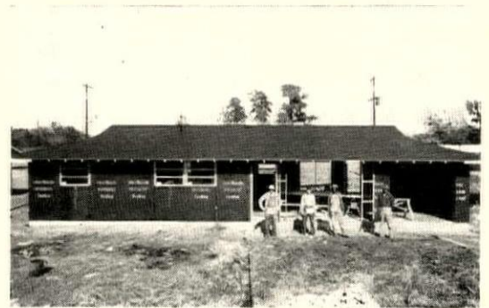
4:30 PM House is completely closed in.
