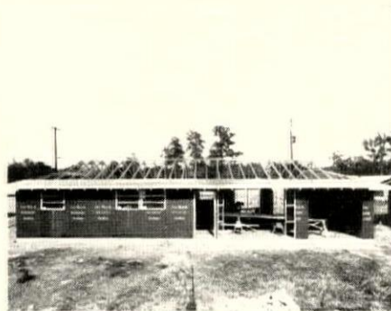
2:30 PM Sheathing is nailed to trusses.
