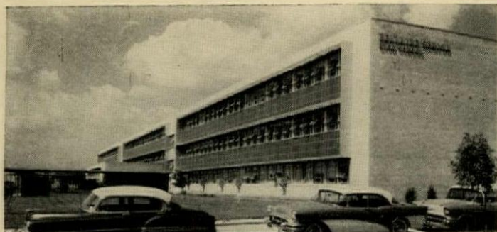
HIGH SCHOOL in Bellaire is typical of schools built by city.
