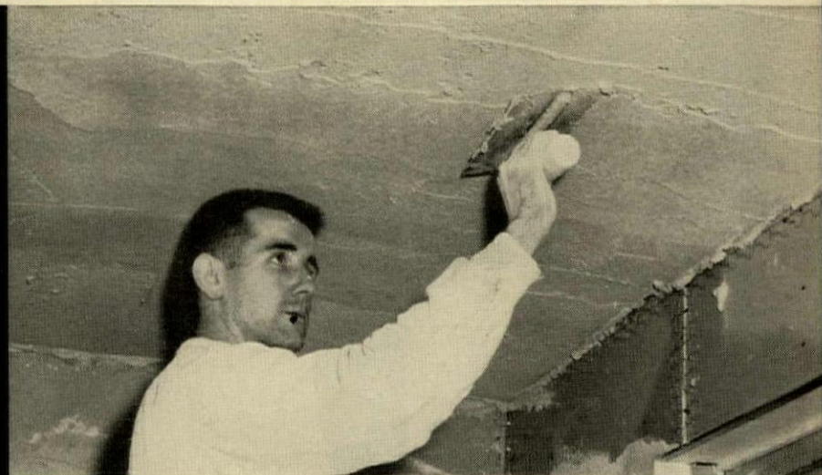
Plaster is applied over reinforced ceiling. The open mesh of both Keymesh and Keycorner assures imbedment in plaster. The open mesh also insures full bond of plaster with gypsum lath.
