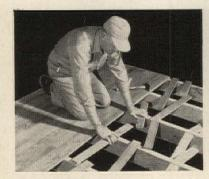
Typical time-consuming assembly job with odd lengths and shorts found in conventional flooring.
