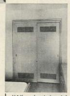
H&K perforated metal grilles in closet doors allow free circulation of air.
