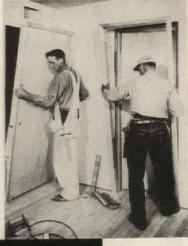
Simply slip the halves together in the opening and nail it in place
