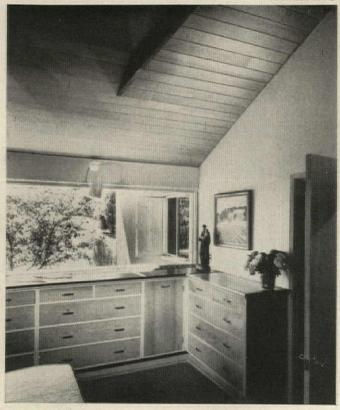
**MASTER BEDROOM** (c) has luxurious built-in storage. The counter surface over drawers has slate top. Cathedral ceiling is clapboard with rafters as in living room (below). Deep lintel over window allows unbroken expanse of glass (see drawing, p. 145). Bath (at right) is private.
