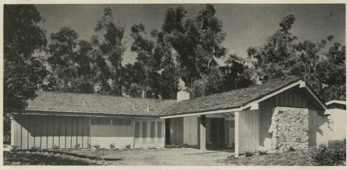
FRONT VIEW shows shake roof, reverse board-and-batten siding, stucco under windows, louvered doors to air conditioner, stone at end of carport.
