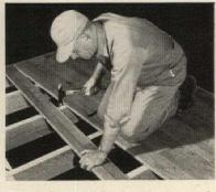
Ease of assembly, drawing-up and nailing MICRO-MATCH is illustrated above
