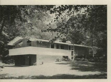
**SPLIT-LEVEL ENTRY**, reached by path from driveway, is between first and second floors, gives equal access to both. From entry, exterior plywood panels with battens extend around house to form balcony wall (left). Other siding is 6" t&g fir. First-floor walls are cement block.
