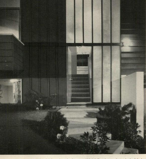
PLASTIC PANELS in a 2x4 frame dramatize the entry, which is halfway between the two levels of the house.
