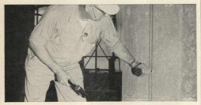
Johnson Service Co., temperature control installers, anchor twin control tubing with Shure-Ser. Drives into hard concrete without a cartridge.
