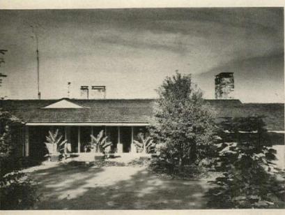
FRONT ENTRANCE (at left) and row of windows are protected by 8' overhang. Windows are in dining and kitchen area, which is three steps below outside grade to let house fit into hillside. Small gable breaks roof line, is repeated on far side of house over living room.
