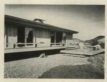
ON VIEW SIDE, the wall is mostly sliding glass doors. Upper deck runs the full length of the house; lower deck is outside living room only. Canted fascia makes a thin roof edge (see drawings on pp. 88-9).
