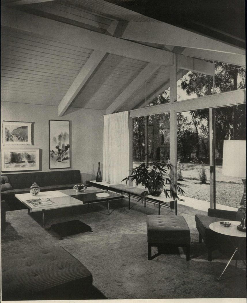
Builder: Schwartz-Yedor Building Corp. Architect: John C. Lindsay, Location: Santa Ana, Calif. beam, do not butt into it (see drawing, p. 156). Ridge beam is carried on 4x6 post in center of end wall. Fir ceiling continues beyond gable to form soffit. Room is vented by jalousies behind curtains, left.
