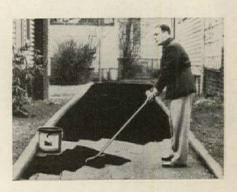
q. Driveway topping and sealer combines the resilience af asphalt with the hardness of tar, won't soften in hot weather or crack in cold weather. Use this liquid patch just as it comes from the container. It dries to a hard luster in two to three hours. Product resists gasoline and grease, completely waterproofs and seals driveway at minimum application cost, maker says. One gal. (\$1.75) covers 50 to 60 sq. ft. Sylvania Chemical Co., Cleveland.
