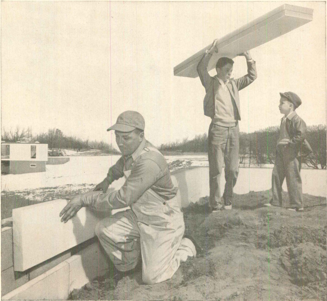
Perimeter Insulation —Wolfe & Gilchrist recommends Styrofoam for perimeter insulation in all their homes. Here Styrofoam is used in Detroit suburb to assure lifetime of warm floors and lower fuel bills.
