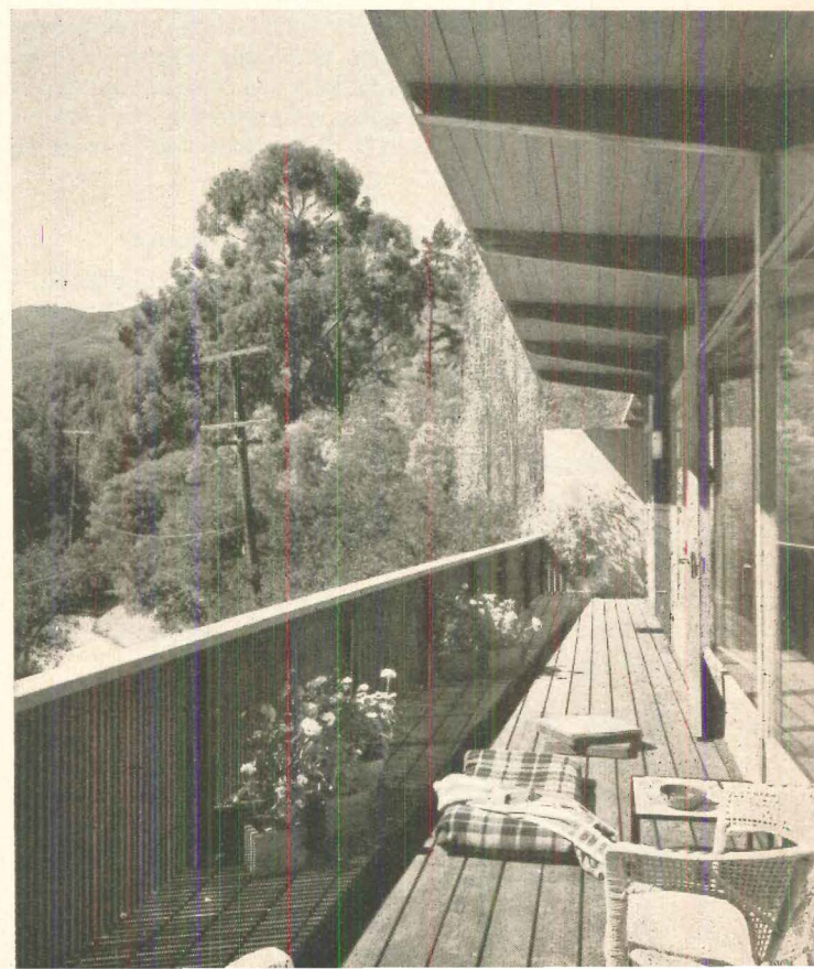
A 55' LONG WOODEN DECK overlooks valley, wraps around two sides of house. Projecting wall panel at far end screens deck from the main entrance./END.
