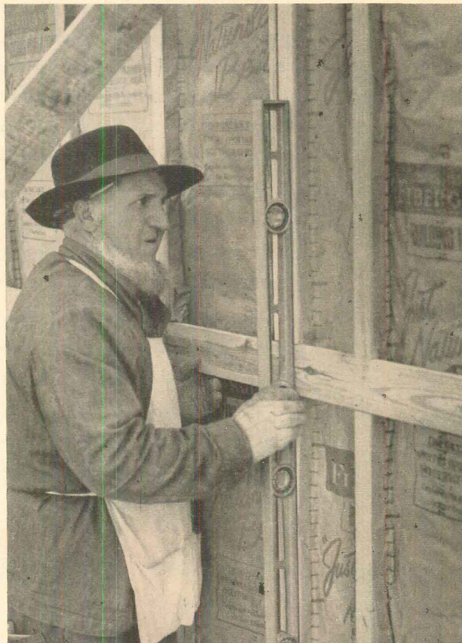
EXTRA RIGIDITY —Note how 1" x 4" half-stud on one edge of panel joins 2" x 4" stud on next panel to make a 3" x 4" support every 4 feet. Notched-in 1" x 4" nailing-strip across mid panel is another American Houses' extra feature.
