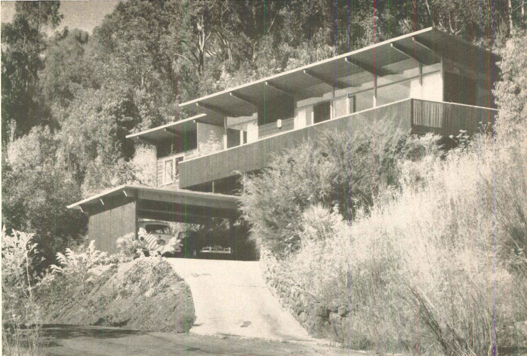
DRIVE-THROUGH CARPORT on lower level is wide enough to take two cars. Low parapet upstairs assures privacy for living areas.
