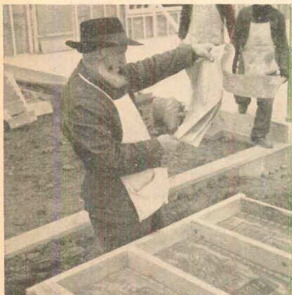
UNITITE PANELS —Basic element of American Houses' construction is the 4' x 8' Unitite Wall Panel, ready-to-erect with insulation in place.
