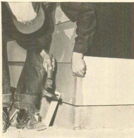
5 Neat, trouble-free corner construction is easy with Duraply lap siding. Special aluminum corners are a snap to install quickly, cost only pennies extra. Duraply superiority is seen in the number of "repeat" orders builders have made.
