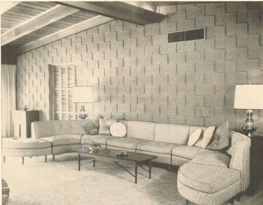
Concrete brick with extruded mortar joints and long low split units combined in this ranch type home.
