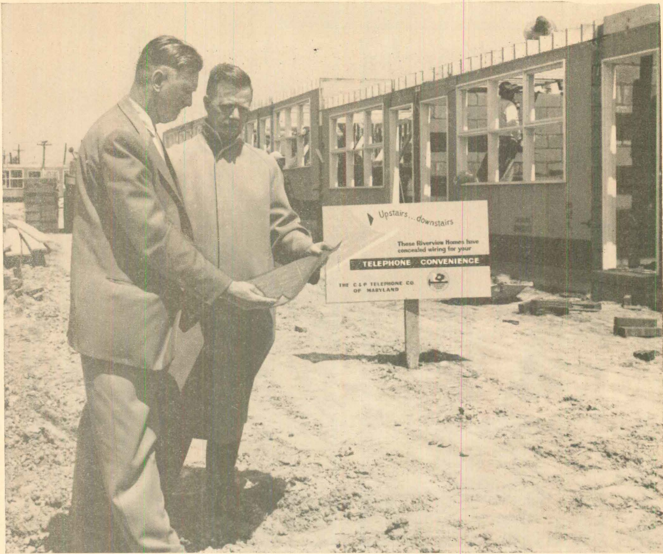
Mr. Knott (right) at the location of his Riverview Homes project in southwest Baltimore, Md., with Earl Schultz, Sr., Construction Superintendent.
