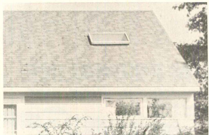
SKYLIGHTS CAN FIT A PITCHED ROOF as well as a flat one. Here is a special pitched roof unit designed to bring light and air into an expansion attic economically. House by Builder Cy Williams.
