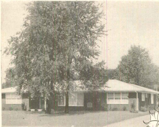
George B. Rice, contractor, easily installed four General Electric "Built-In" Thinline Air Conditioners during construction of this new house at 2105 New Market Drive, Louisville, Kentucky.
