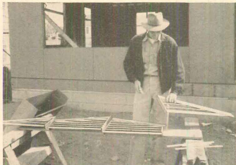
Sections of a large louver are assembled quickly using slip-joint fasteners to hold them together
