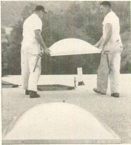
F. Wascolite: single and double shell. Clear or translucent acrylic. Self-flashed curb with or without vents. Wasco Products, Inc. Cambridge 38, Mass.
