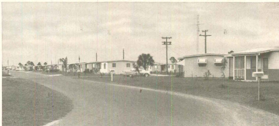
At the Pompano Beach development, 1200 houses have been erected, with L-M Permaline pipe used exclusively for house-to-street sewers. The developer eventually plans to have 2800 homes suitable for retired people on these beautiful highlands near Miami.
