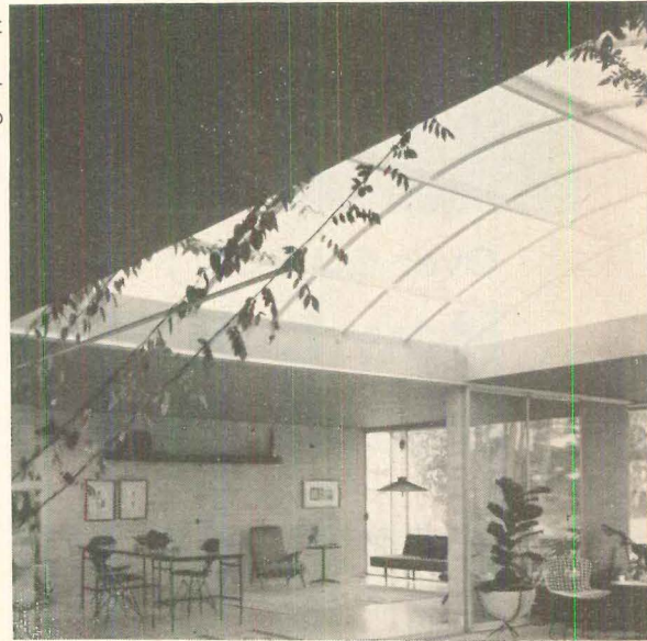
6. CENTER COURT or patio has big span of durable plastic to let in light, keep out rain. House by Architect Paul Rudolph.
