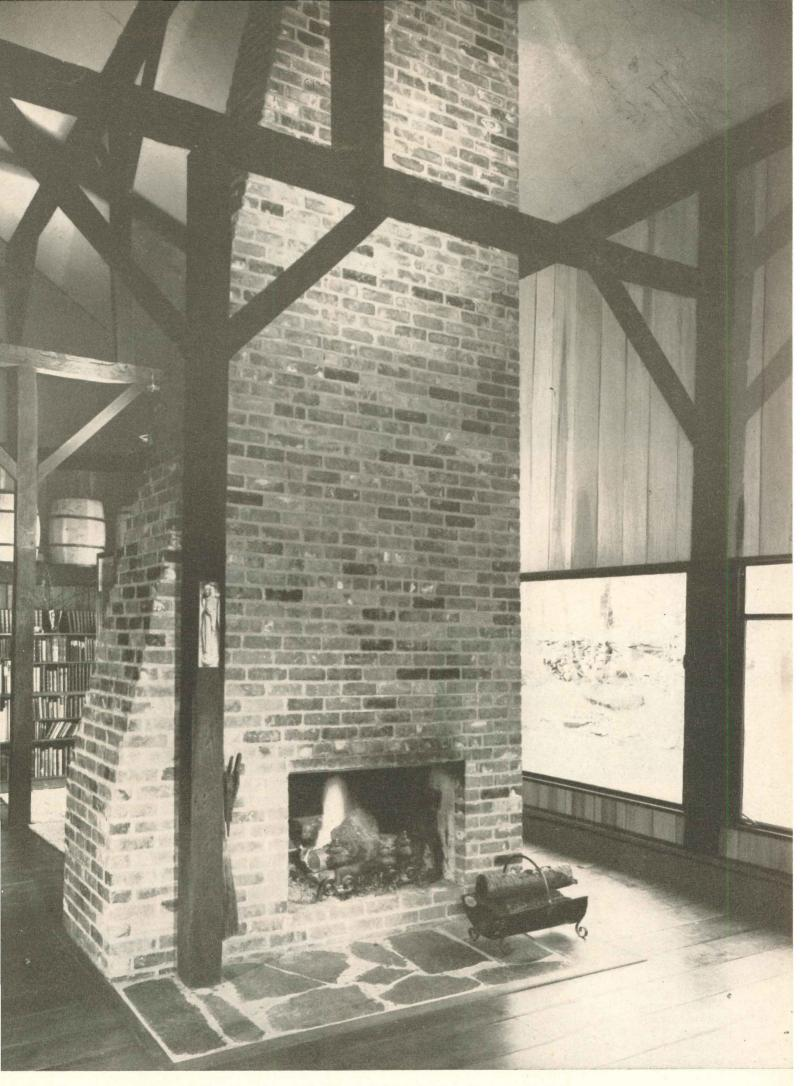
Fireplace chimney rises to ridge pole; room height is emphasized by exposed structural framing
