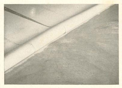
Rolled flooring is applied directly on concrete over new adhesive
