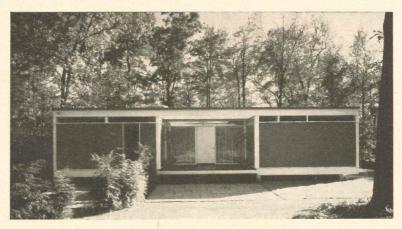
Entrance faces north, is formal, near-symmetrical. Post and dropped beam construction was used throughout. Slots of glass fill in space between ends of beams.
