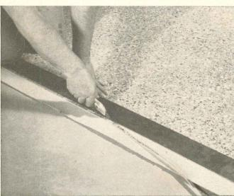
Edges are cut and trimmed with straight blade knife
