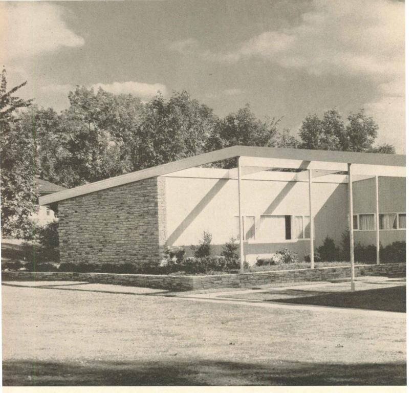
Pitched roof trellis over entrance court is supported on two rows of lally columns—one running along ridge line, the other offset
