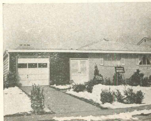
From street, patio is not visible, unusual privacy for Long Island.
