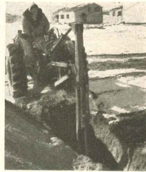
Small backhoe trencher digs sewer lines on sites.
