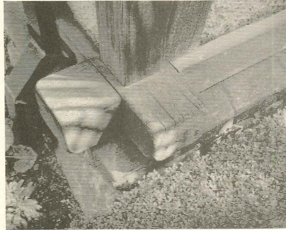
Post and plates interlock at corners
