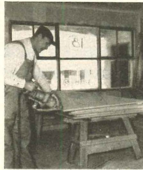
Portable power saw is basic tool on L.I. projects.
