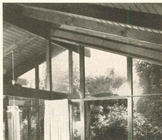
Exposed beam ceiling with plank deck
