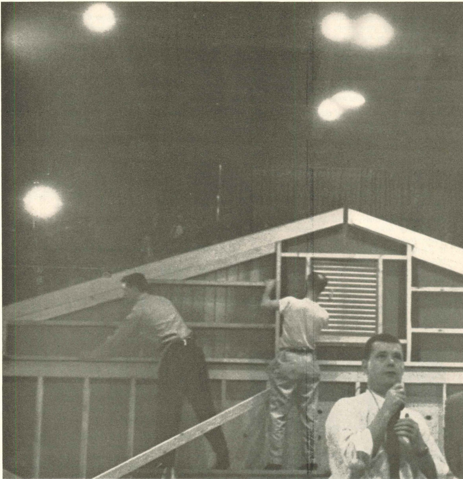
Upside down trusses are hung on framing, then tipped into place.
