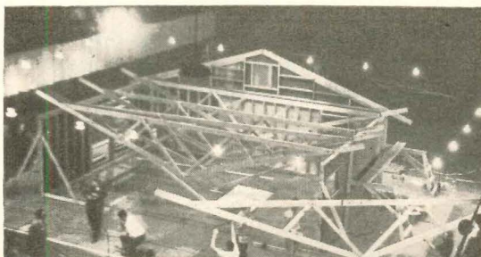
Upside down trusses are hung on framing, then tipped into place.
