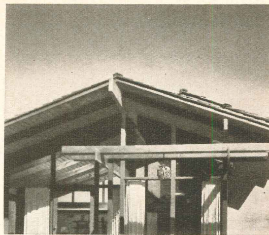
New gable end has projecting rafters also
