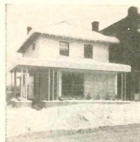
Old house (left above) was remodeled for offices (left) in 1951 by Haverstick firm, then rebuilt into handsome offices below. Ground floor and basement are rented. So Joe enjoys his second-floor almost rent free.
