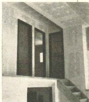
Drywall in splits must fit around many small surfaces.
