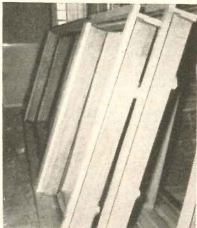
Prefabbed windows are of structural millwork.
