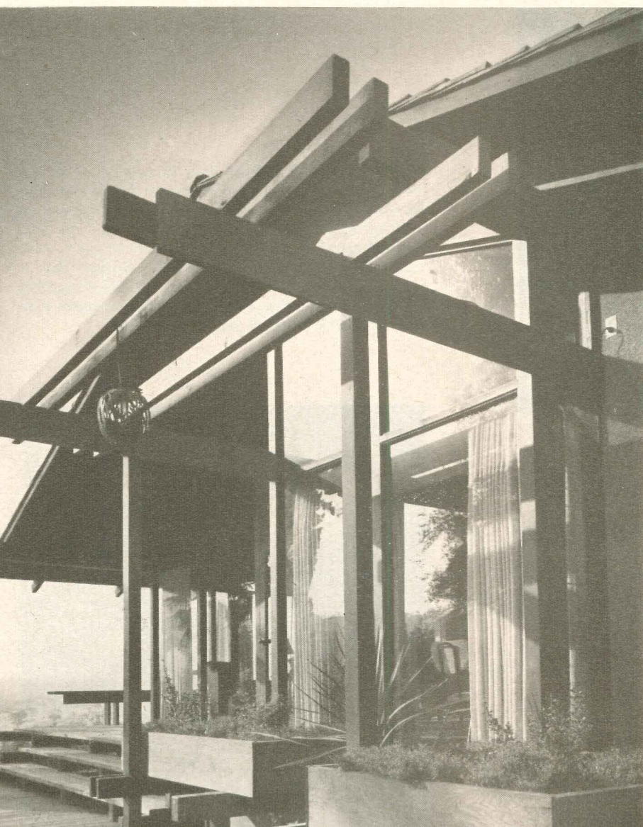
Footings carry interlocking post and beam frames
