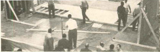
Coliseum floor serves as nailing platform for 24' gable end wall.
