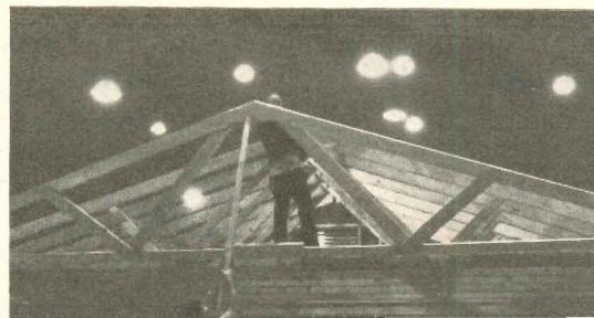
Agile workman spaces trusses, as others spike truss heels to plate.
