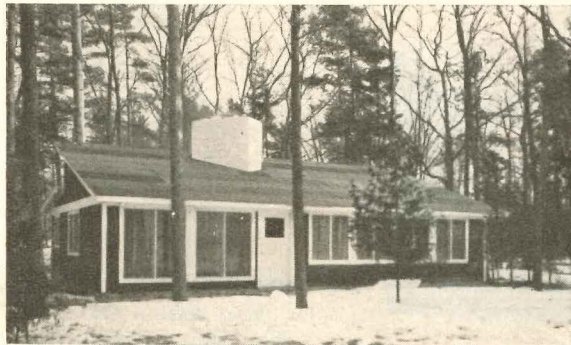
Summer cottage in Michigan has lots of wood paneling, was designed by Architect Roland Rosser.
