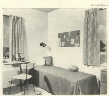
Flat, smooth wall surface is result of tape over gypsum
