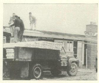
Unloading direct from truck to roof saves valuable handling time. Cumbersome old-style materials have to be dumped on the ground, then hoisted to the roof as needed. Securely wrapped Armstrong Temlok Roof Deck—32 sq. ft. to the package—is easily stacked on a small portion of the roof until it is used.
