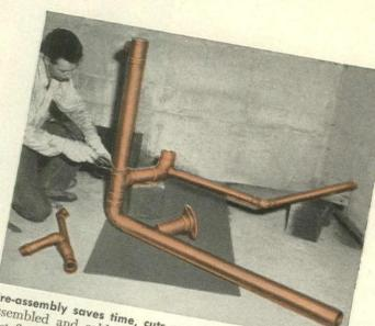
Pre-assembly saves time, cuts cost: The basement lines are assembled and soldered ready for installation as soon as first floor partition studding is completed.
