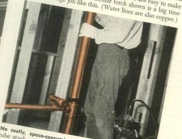
Write for booklet, "Copper Tubes for Sanitary Drainage Systems." The American Brass Company, Waterbury 20, Conn. In Canada: Anaconda American Brass Limited, New Toronto, Ont. No costly, space-consuming plumbing walls: A 3" copper tube stack with fittings can be installed within a standard
