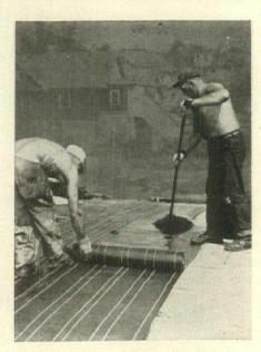
and bond into a solid mass, eliminating one common cause of blistering-felt touching felt. The reinforcing reduces cracking or "alligatoring" of the actual weatherproofing agent, the bitumen. Because the glass fibers are inorganic, they do not rot or deteriorate.
