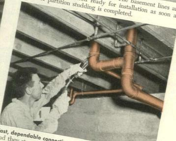
Fast, dependable connections: Solder joints are easy to make and they stay tight. The circular torch shown is a big time saver on a large job like this. (Water lines are also copper.)
