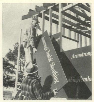
Less waste because Temlok Sheathing fits accurately over framework of studding 16" on centers. Temlok waste is only 5%, compared to an average of 20% with wood. There's no dimensional loss with Temlok—2' x 8' Temlok is full 24" wide, while 6" wood sheathing is only 5%" wide.
