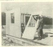
Closest to conventional construction is 2x4 panel (Scholz, Lu-Re-Co) which doubles up studs at panel joints. Most panels are shipped with exterior sheathing applied, sometimes with siding materials already on. Tendency now is to ship panels with interior gypsum ready for taping on site, insulation in and provision made for wiring.
