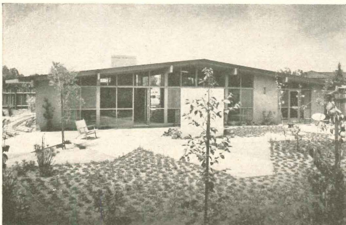
Plan has back-to-back bathrooms, compact kitchen. Water heater and furnace are in closets off front entry, laundry at end of kitchen.
