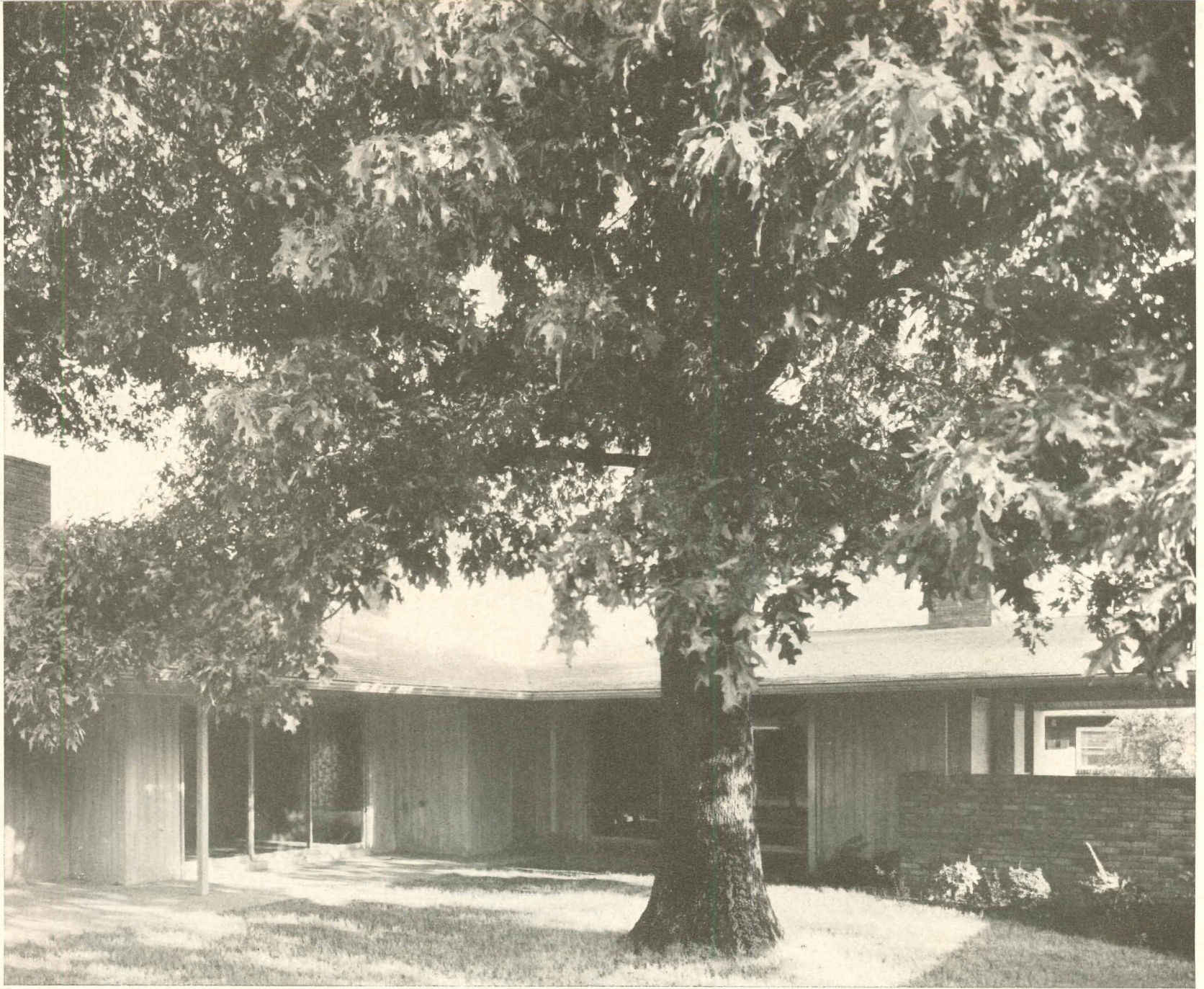
Sliding glass walls toward front garden are protected by deep overhangs, ancient tree
