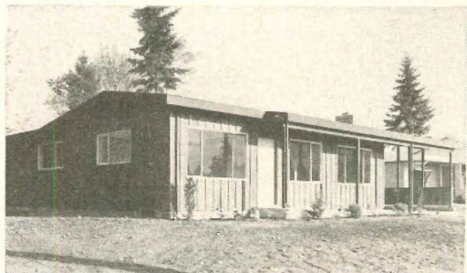
Wide overhang is supported on columns, provides shelter from carport to front entrance.
