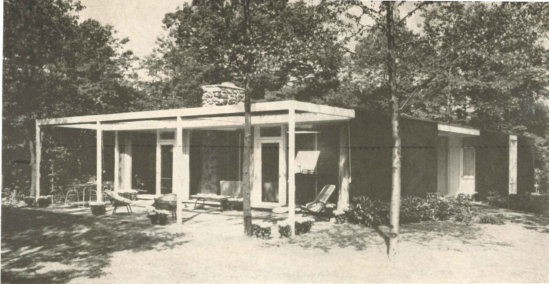
Post-and-beam porch has movable canvas "roof" that can be adjusted to shade the glass wall in the living area
