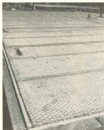
Topping operation using 1/4" concrete over mesh reinforcing was later found necessary.
