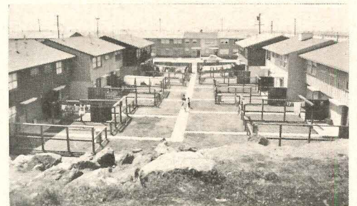
3. Fenced back yards serve as private outdoor living or service areas. Arrangement of row houses creates a series of large courts, each with distinct character of its own. Several open up toward view of hilltop.
