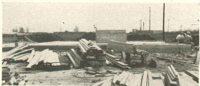
Complete frame at foundation, pre-cut and ready for assembly
