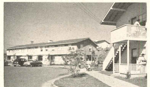
4. Cul-de-sac parking lots reach halfway into groups of houses, bring cars within easy walking distance of all houses. Parking areas act as "space dividers" rather than off-street islands, enlarge distances between rows of houses.
