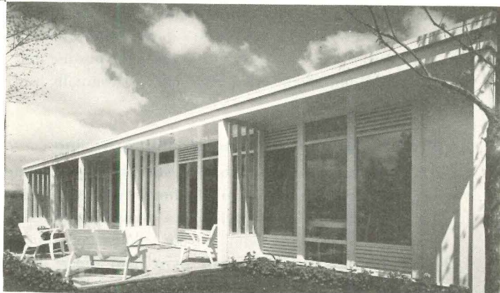
1944: Green prefab, designed by George Fred Keck and William Keck. Modular panels were 3'-3" wide, included louvered ventilating units.
