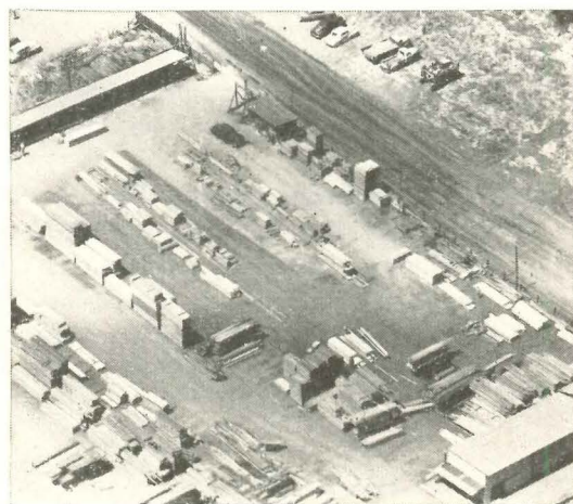
Two loading lines (center) and cutting shed (lower right) in one corner of Wight's San Carlos, Calif. yard are laid out in a U-shaped plan to minimize movement of cut stock, conserve space for inventory.
