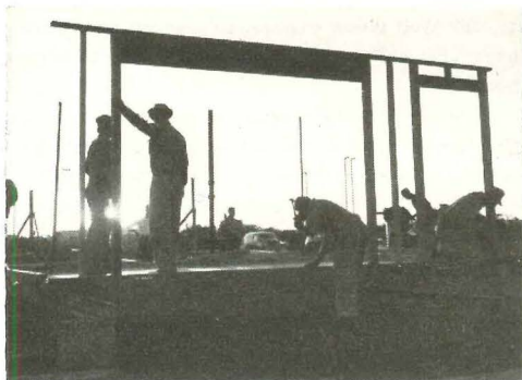
WORKMEN BEGAN HOUSE-IN-DAY AT DAWN
