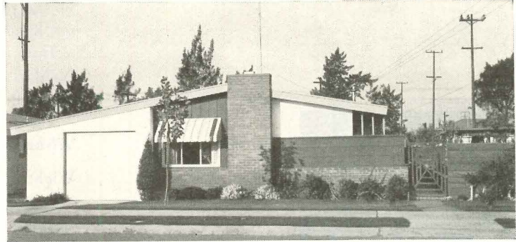
Pittsburgh Construction Co., builders. Location: Pittsburgh, Calif.
