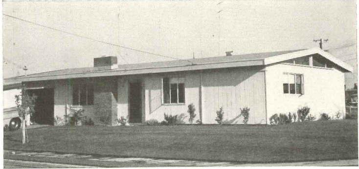
Triad Construction Co., builders. Location: Antioch, Calif.
