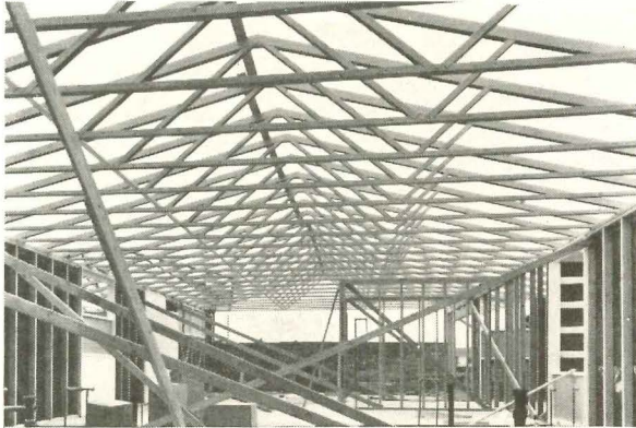
Steel trusses by Ned Cole span 24', weigh 110 lbs. each; can be fully dismantled for fast, inexpensive shipping.
