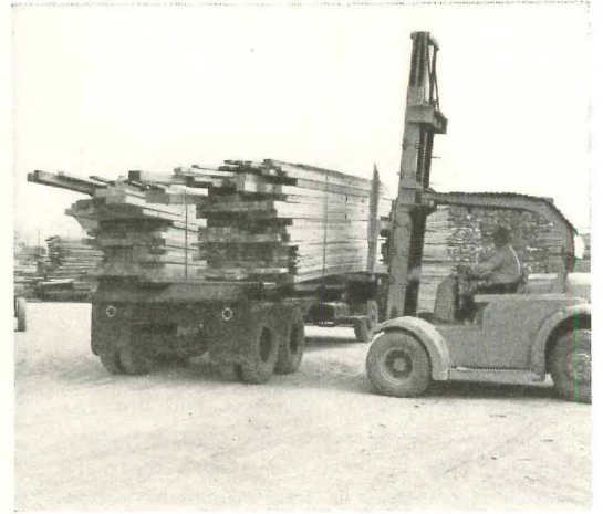
Steel-strapped packages are loaded two to a truck ready for delivery to site. "Handling and loading," says Wight, "are as important as production-line cutting operation in achieving lumber economies."
