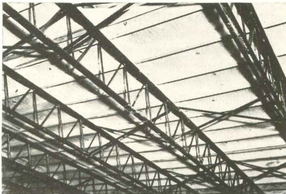
Steel floor joists by Modern Homes are 180 lb. each, 24' or 28' long, 24" o.c., can be set in place by two men.
