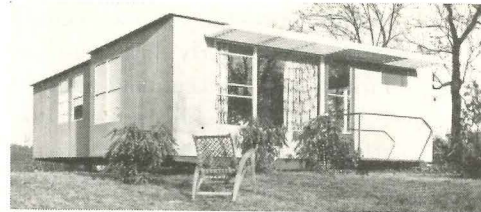
1948: Acorn House, designed by Carl Koch. Entire house folds around utility core for compact shipping on trailer truck, unfolds again on site.
