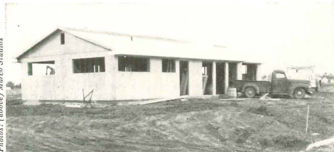
At 3 p.m. house was this far along, and by 5 p.m. was closed, windows and doors hung, siding and roof papered.
