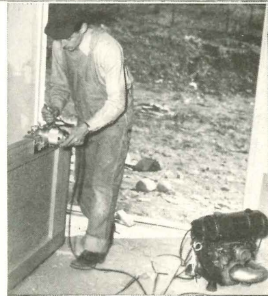
Machines like this one in National's Lafayette (Ind.) plant result from prefabber's ingenuity. In 15 seconds, it mortises and drills all holes needed in a door—formerly a 12-minute operation. Conventional builders can gain greater efficiency for same operation by using electric combination router-planer (right) to trim doors, mortise and make butt joints.
