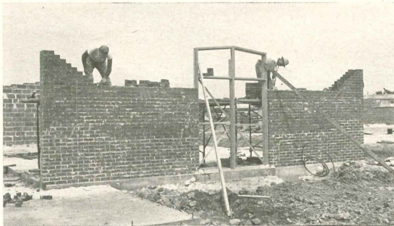
Simplified scheduling is made possible by concentrating brickwork in vertical "panels" (photo). Redwood siding on long-side elevation (left) is neatly framed between 10"-thick brick cavity walls, avoids abrupt appearance usually seen in brick-and-wood houses.
