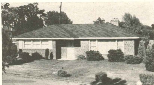
1947-48: first subdivision of 30 houses, Maryknoll, was built when young builders had trouble getting suitable lots. Noting how high building costs squeezed down room sizes, they decided to build basementless houses with radiant heat. Hip-roof house of brick sold for $9,500, had 1,150 sq. ft. Note size of picture window in front.
