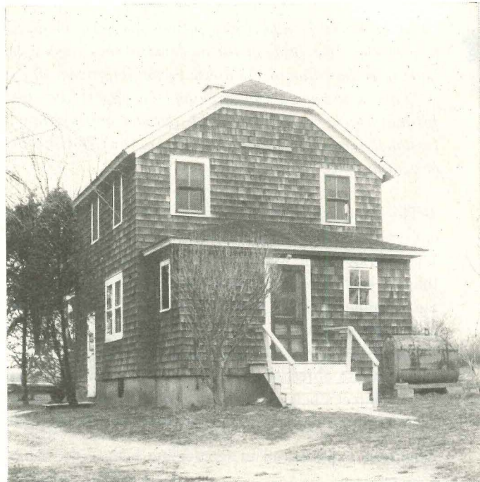
Before: chief access to back yard was through kitchen porch
