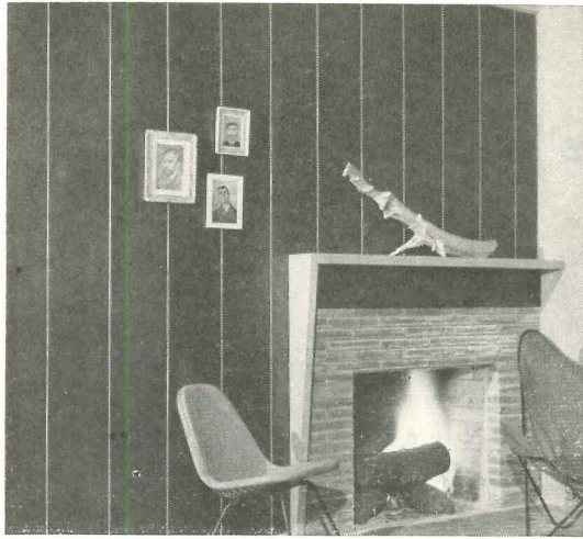
Harborite panels put resin face forward in interior use, are painted when used on exterior.
