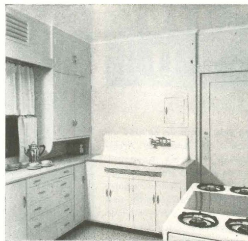
After. Wheeler also put new plywood fronts on cabinets and undersink radiator, raised counter to sink's height, provided toe space. New linoleum, paint, and breakfast alcove brought cost to less than $500.
