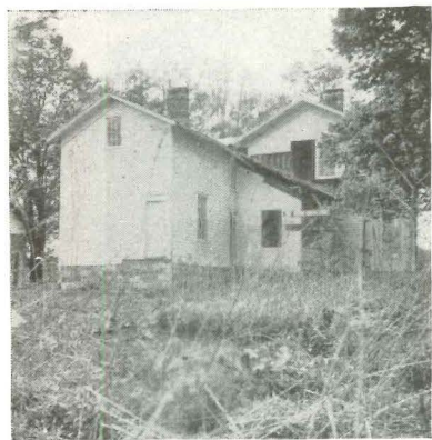
Before: old lean-to contained a woodshed and attic.
