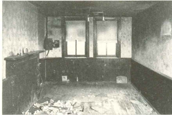
Before. Heavy, dark trim in old dining room made it seem small, oppressive. Remodeler Mrs. Una Hanbury removed part of chimney, used bricks on floor.
