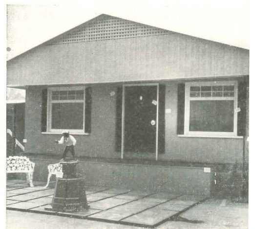
After it moved to the used-house lot, house got the lifting. Foundation is temporary.
