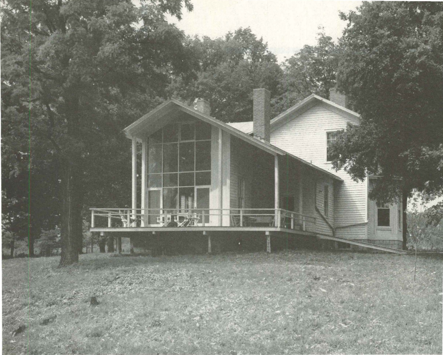
After: two-story living room and porch now face the garden and overlook a lake. Cost of remodeling the old woodshed alone was $5,000. Additional $7 spent on rest of house, especially bedroom areas.
