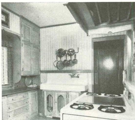
Before. Remodeler W. S. Wheeler of Minneapolis covered badly cracked ceiling with wood-fiber insulating tile board for $53, saving costly replastering job, removed fake range hood, put a vent fan in outside wall.
