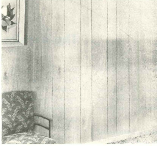
Balura has imported hardwood face over economical core of less-costly native woods.
