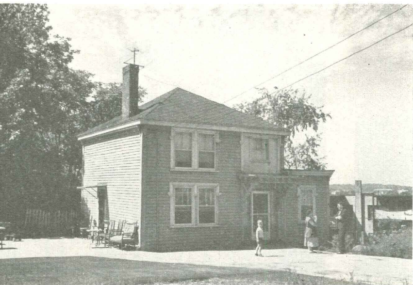
Run down and in a poor neighborhood, old house (left) had so little market value Turchon found a do-it-yourself owner, a maintenance man who paid only $250 down, total of $5,600. Turchon's carpenter helped with work which included turning two small rooms into a large room, new aluminum windows, new ceilings, linoleum floors, new kitchen and bath, all new paper and paint. Lot is over one acre. A Boston bank took a conventional mortgage.
