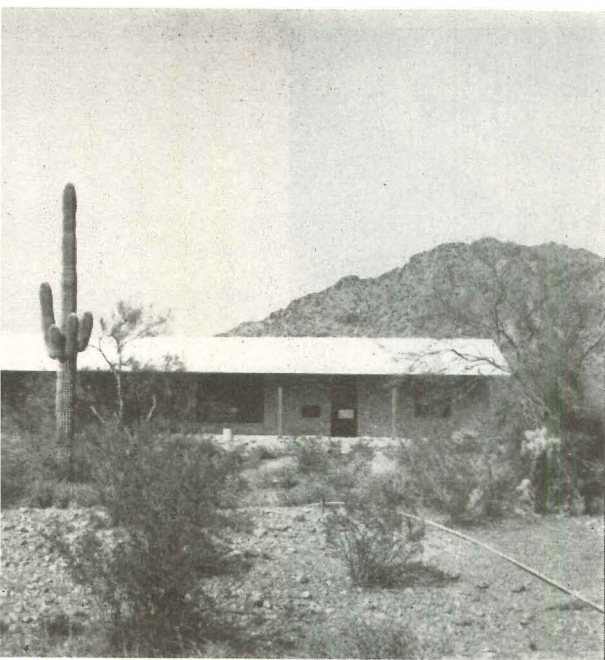
House of Kenneth Sloan outside Phoenix was designed for window air conditioners, with two 1-hp units in living room, one in each bedroom, and one 3/4-hp unit in each of two bedrooms. He specified window units instead of central unit because they gave him flexibility of control. Only room cooled is a room being occupied.
