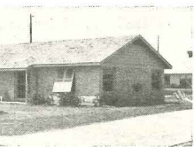
15, 1,248 under rafters, ulation, ilating fan s, s on southeast ard sheathing, asterboard
