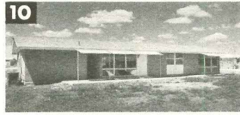
10 S. R. Sheppard; 1,300 aluminum foil under rafters 4" ceiling insulation 36" overhangs, part double glazing, canvas awnings on southwest 2-ply foil 22,891 Frigidaire
