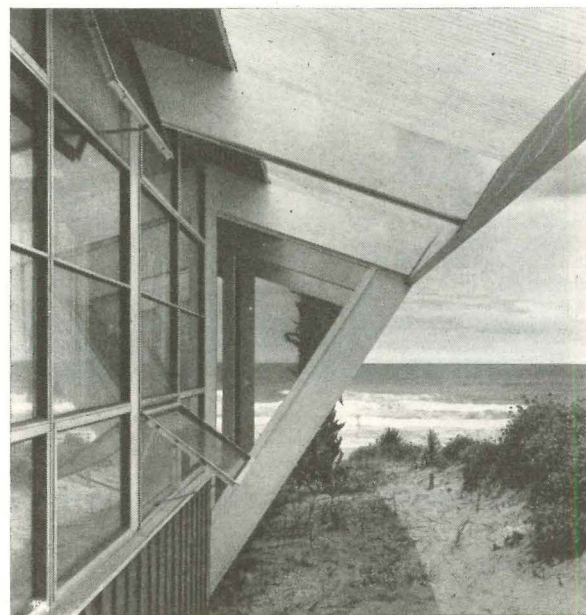
Corrugated plastic , reinforced with glass fibers, forms overhangs that keep off rain and sun but let in light. Over south side (above and below) is a 36' strip cut from 100' roll, green in color to "cool off" harsh sun before rays enter kitchen and dining room. On the north a 50' length of yellow plastic lets in a warmer light.
