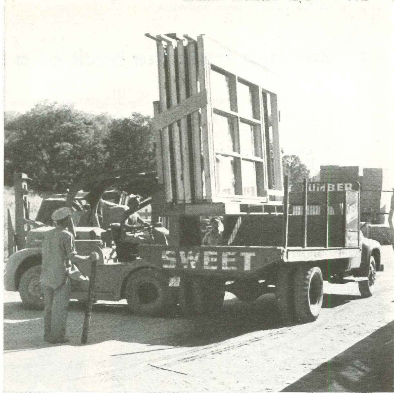
Completely sided and insulated, panels are lifted into delivery truck
