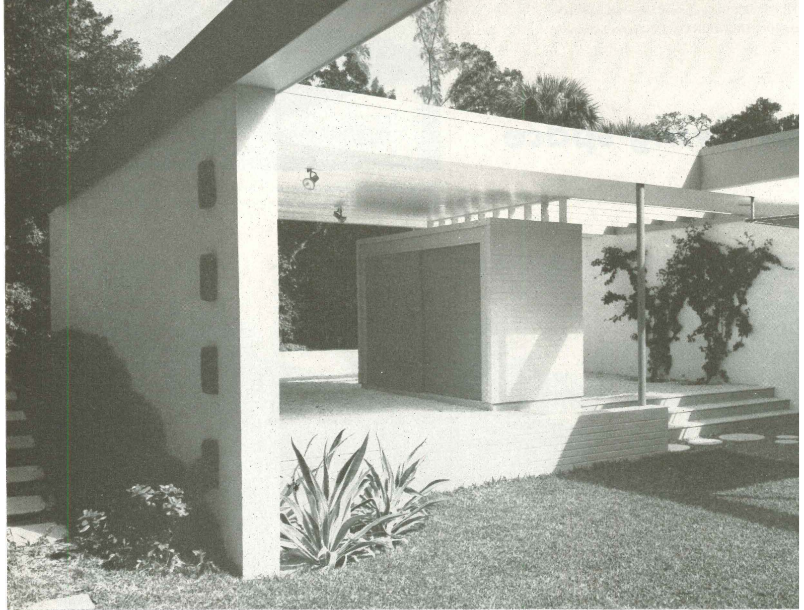
Carport at left, outdoor foyer at right. Note glimpse of living patio through front door of house
