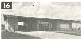
16 H. T. Baker; 1,390 3" rigid insulation, in pitched, built-up roof 36" overhangs, outside awnings 4" insulation 25,288 Lennox
