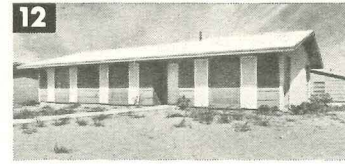
12 B. N. Holman; 1,250 6" ceiling insulation 36" overhangs, reflective screening insulation board sheathing, 3/4" rigid insulation, foil-backed plasterboard 26,017 American Furnace
