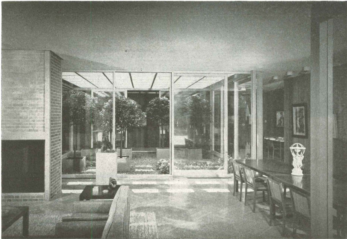
Floors are of Sicilian travertine throughout. Its color is that of wild honey. Steel was painted taupe
