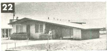
22 W. H. Bullard; 1,200 6" ceiling insulation 30" overhangs, reflective screening 2-ply foil 24,080 General Electric
