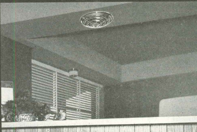
Austin Air Conditioned Home #11, built by Frank Barron, includes a NuTone 829 Ceiling Ventilating Fan in center of the kitchen.
