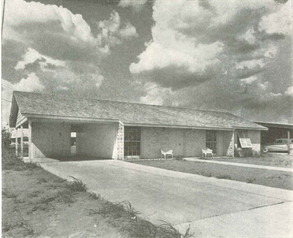
Vertical shading devices next to windows, like these two ornamental iron grilles, can be effective in reducing direct sun on windows. Late afternoon sun is often so low in the sky it gets under the widest overhang. At extreme right (above) is a louvered wood shutter.
