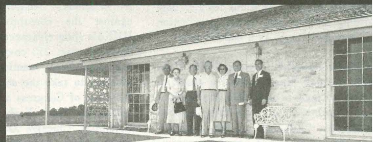
NAHB Air Conditioned Homes #6 and #12, built by B. N. Holm, equipped with NuTone Model 821 Ceiling Ventilating Fans in the living room and bedroom.
