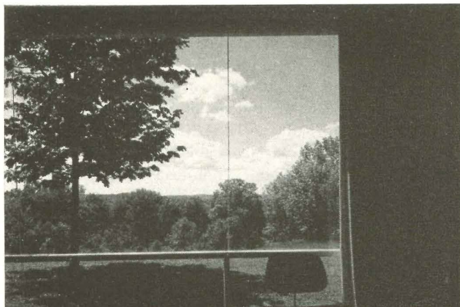
Louvered metal insect screening is a shading device, which manufacturer says lets only 12.5 to 18% of sun heat enter the room. Designed like miniature Venetian blinds, these screens let in light, but greatly reduce glare and will help to reduce the load on air-conditioning equipment. Such screens are made to fit any type of window.
