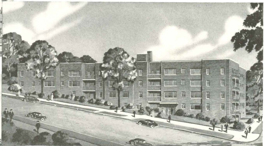
The ultra-modern Carlton Terrace in Bronxville, New York.
