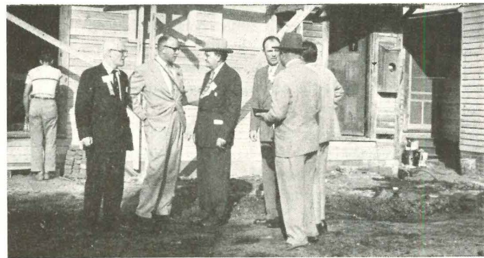
REHABILITATION pilot project on New Orleans' Conti St. was visited by NAHB bigwigs including (l to r) Joseph Merion Alan Brockbank, R. G. Hughes, Fritz Burns, and (backs to camera) Yates Cook and Col. Shelton Hubbard (with hat). Hubbard, 59, took over from Cook as director of the city's rehabilitation department. Hubbard is former director of street sanitation for New Orleans.
