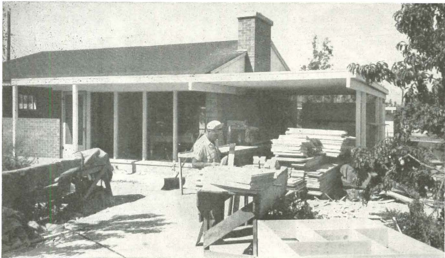
Storage walls are prebuilt and sanded in builders' own shop on project, hauled in sections to each house. Builder Ed Holmes, who has four sons in his family, became sold on the storage-wall idea after putting them in a house built for himself.
