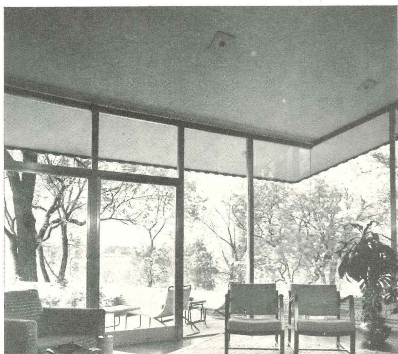
The big view across the lake comes last. Here the living room flows out through glass doors to the planted apex of its terrace. Mitred glass liberates the corner.
