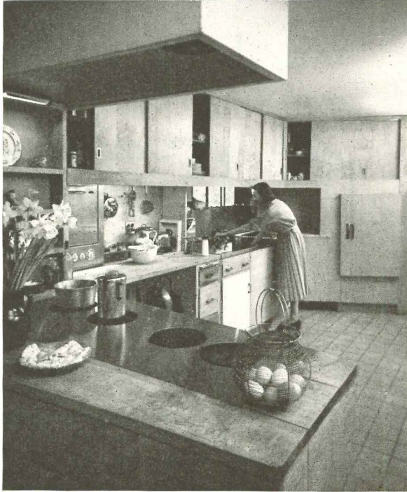
Big hood over range traps heat and odors until exhaust fan can pull them outdoors. In air-conditioned houses housewife should turn on fan only when cooking, be sure to turn it off after cooking.
