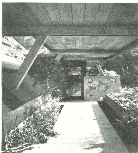
Entry walk is sheltered by a deck canopy cantilevered out from the roof structure. Path is merely an extension of the floor slab inside.
