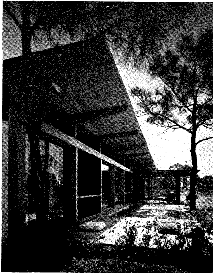
South overhang fully shades window wall in Florida, by Architects Twitchell & Rudolph.
