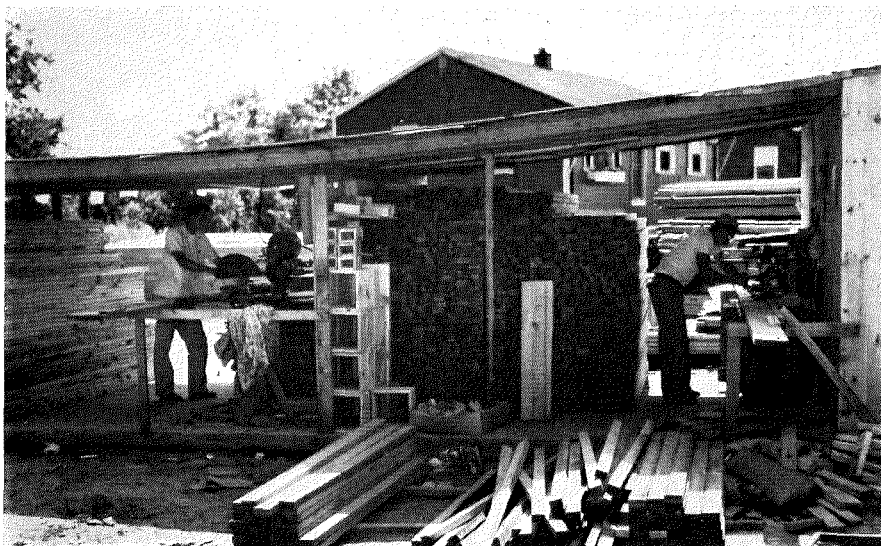
To give the most house for the least money, Bent and Stevens applied many of the labor and materials saving techniques recommended by the Small Homes Council of the University of Illinois. First and foremost: precutting. Virtually every piece of lumber was cut in advance in this special carpentry shop set up on the site, protected from rain.
