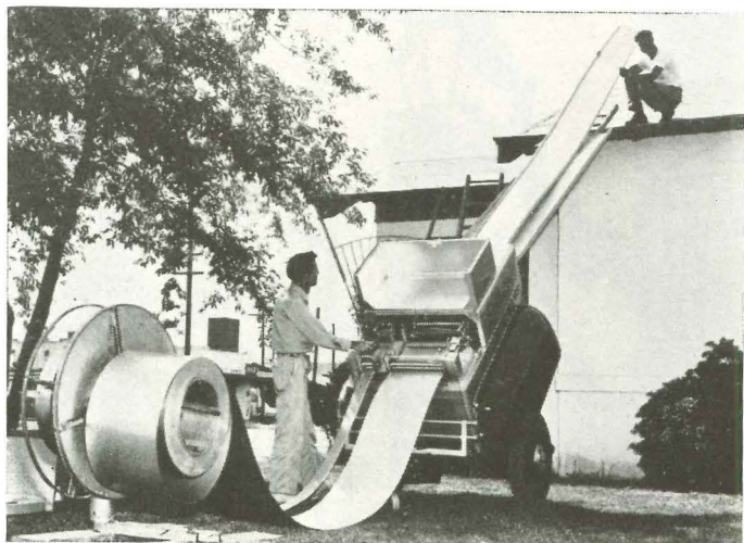
Aluminum pans are directed to workmen on the roof from the two-wheeled former. Clips and battens dress the edges.
