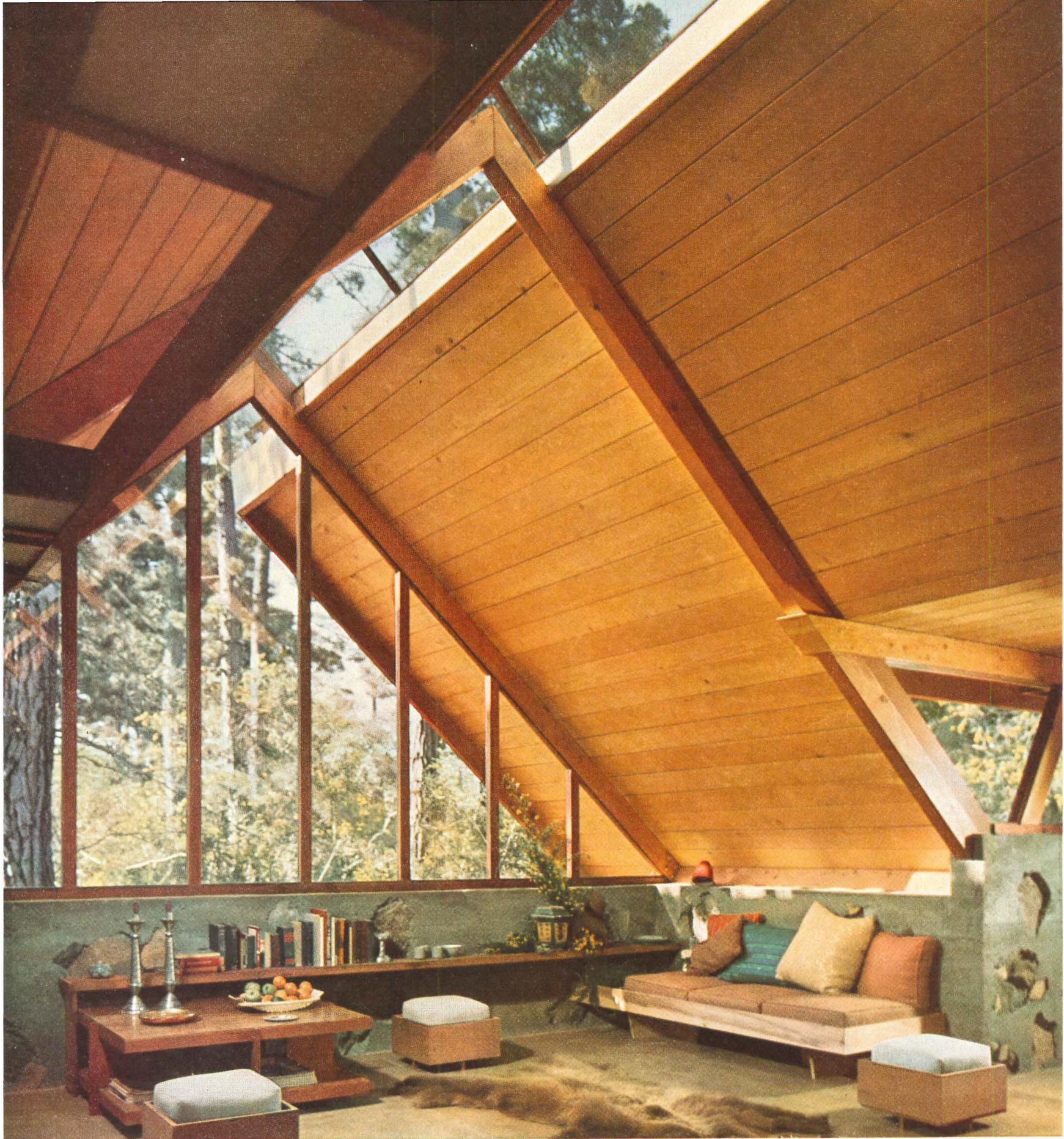
Big tent of wood and glass shuts out the busy street and hot sun on the west, right, opens up the living room to the south through a gable end of glass. The long skylight at the ridge allows the whole house to reach up for overhead light from its dense woodland site. Foundations are of cast concrete masonry—big rocks placed in the forms during pouring. This wall was continued 3' above the ground to buttress the outward thrust of the roof deck, which is bent up to give headroom for an entry hall (right). Floor is a 3" concrete slab, integrally colored and polished to a smooth finish.
