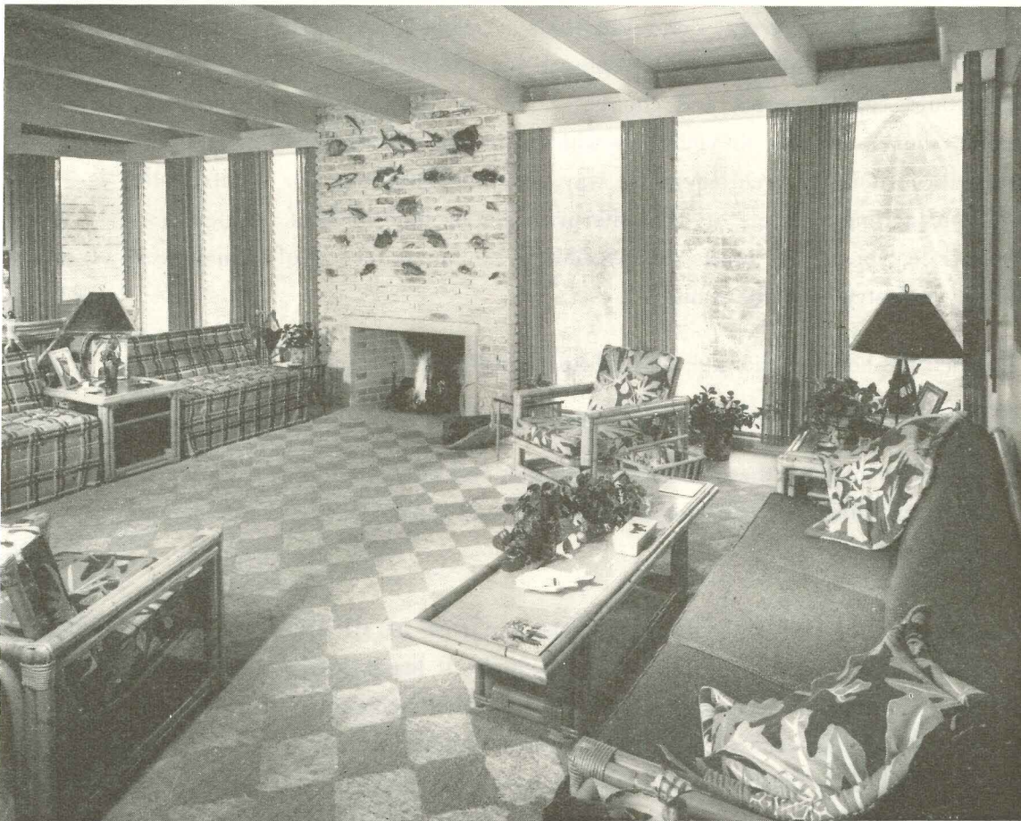
Jalousie windows , seen here in living room, give floor-to-ceiling ventilation, can be adjusted closely for amount of breeze desired, even left open during rain. Insect screening is fitted to inside of windows. Upstairs floors are terrazzo.
