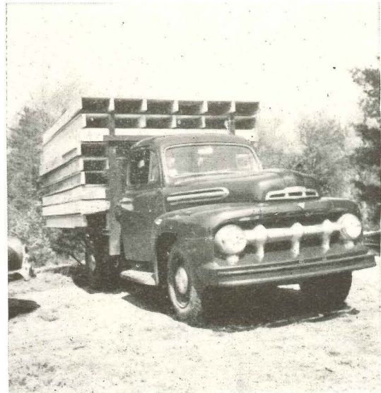
1. Preassembled panels are trucked to site as soon as the foundations are ready. Techbuilt, Inc. currently ships and builds within a 20-mile radius of Boston.
