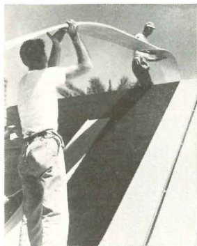
Aluminum pans are directed to workmen on the roof from the two-wheeled former. Clips and battens dress the edges.
