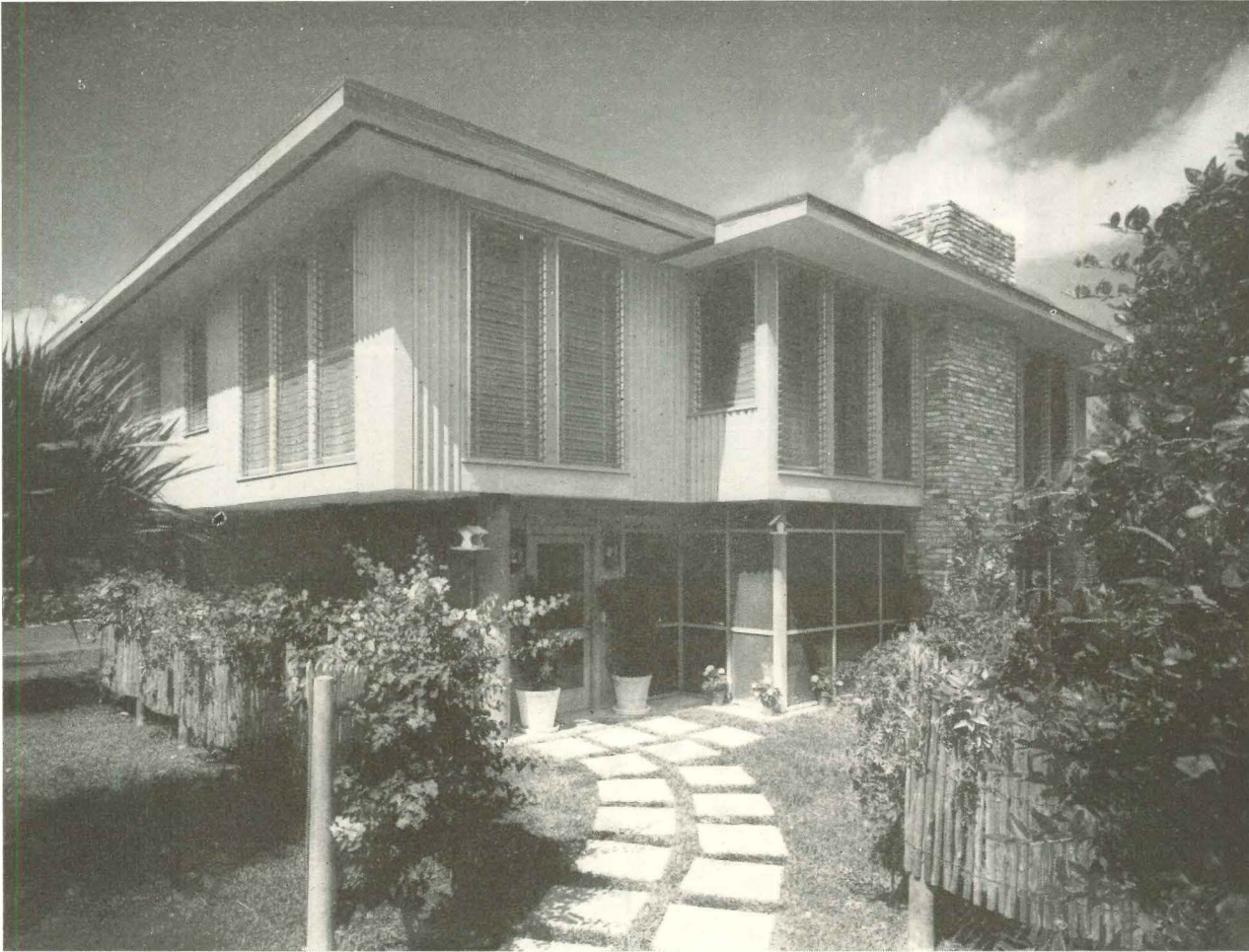
On the entrance side, living room and master bedroom face south-east to the prevailing breeze and an unobstructed view of the bay.
