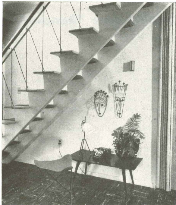
Most novel change in new house is open stairway which hangs like a piece of wall furniture, does not stop the eye as would a closed-in stairwell. Cord lacing in place of wood balusters adds clean, contemporary touch. Stair risers, with clear finish shown here, are now painted in all houses.
