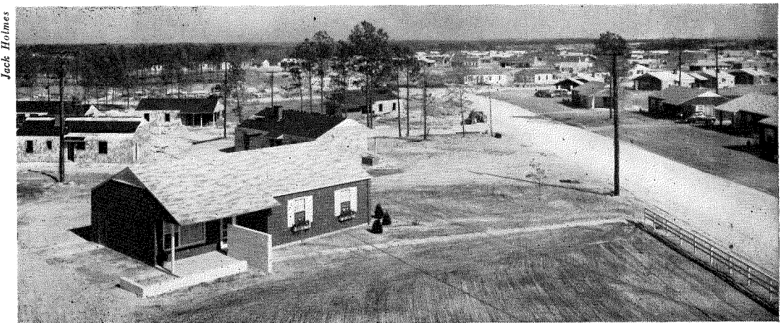
SINGLE-FAMILY HOUSES ERECTED FOR AEC WORKERS IN AIKEN, S. C. BY GROSS-MORTON
