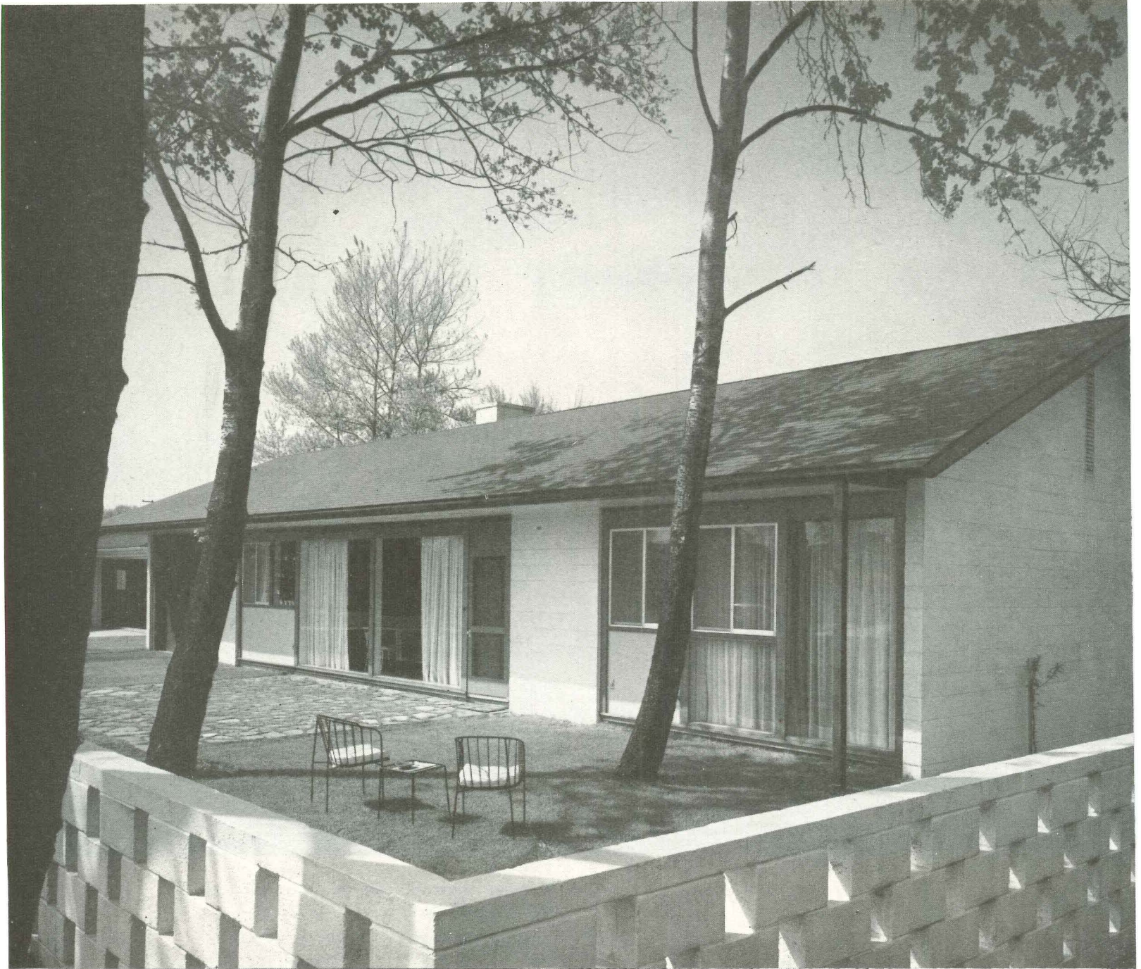
Privacy is assured by placing house 85' back from street behind 4' wall which encloses south-facing terrace. This wall, of standard cinder block laid 6" apart for pattern effect, lets breezes through, has the same effect as a window sill—outside the house—for the “open” floor-to-ceiling glass.
