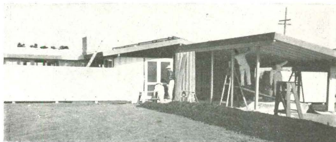
4 P.M. Roof finished, fences up, shell completed
