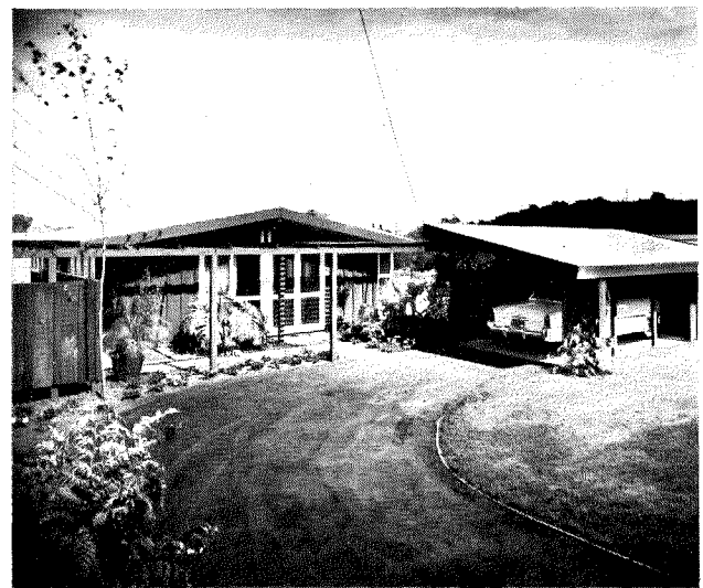
Carports were completely redesigned in new houses and were given sloping roofs to harmonize better with houses. This is the house at Vista in which all the color and interior photos were made. Curved drive is popular.
