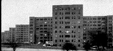
in MULTI APARTMENT UNITS Hunting Tower Apartments, Alexandria, Va. C. H. Tompkins Co., Washington D. C. Con- tractor.
