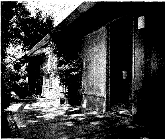
1. Obscure glass shields entry and hall from street
