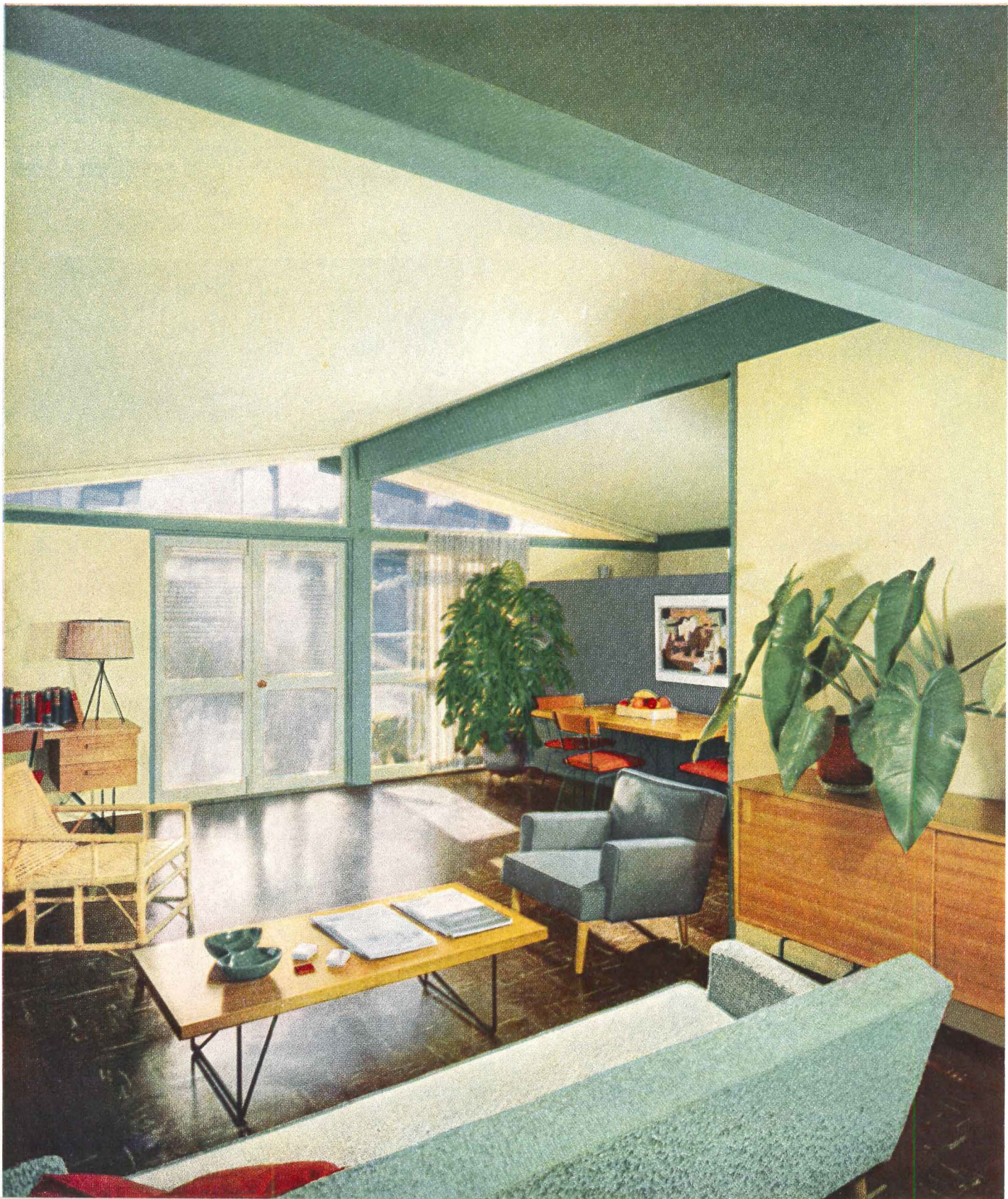
Contrasting colors, below, give decorative impact by emphasizing structure. Three typical panels are in far wall: solid panel with plasterboard interior, pair of double doors, window wall. Glass gable is installed at each end.
