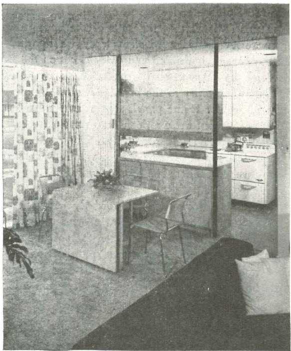
Open kitchen has efficient U-plan, plenty of continuous counter space, big windows up to top plate with view of front terrace and approach. Cabinet above pass-through has sliding hard board doors on both sides, hangs on black angle-iron posts. Stock folding partition, left, closes kitchen off.
