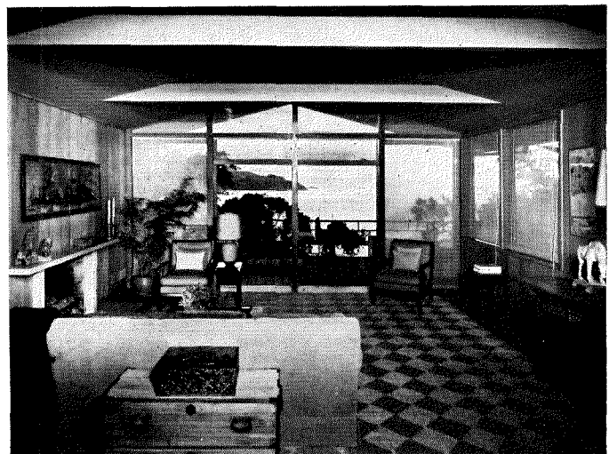
Three arches of doubled 2 x 10's and tie beams carry living room's open ceiling. Trussed 2 x 6 rafters (above) roof bedroom wing.
