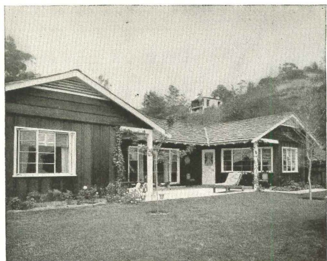
Mr. William A. Zeh, builder of this house at Los Angeles, Cal., says, "No builder nowadays would think of installing anything but automatic heat and electric refrigerators in his new houses. And just as people take those things for granted, they're looking for automatic electric cooking equipment."
