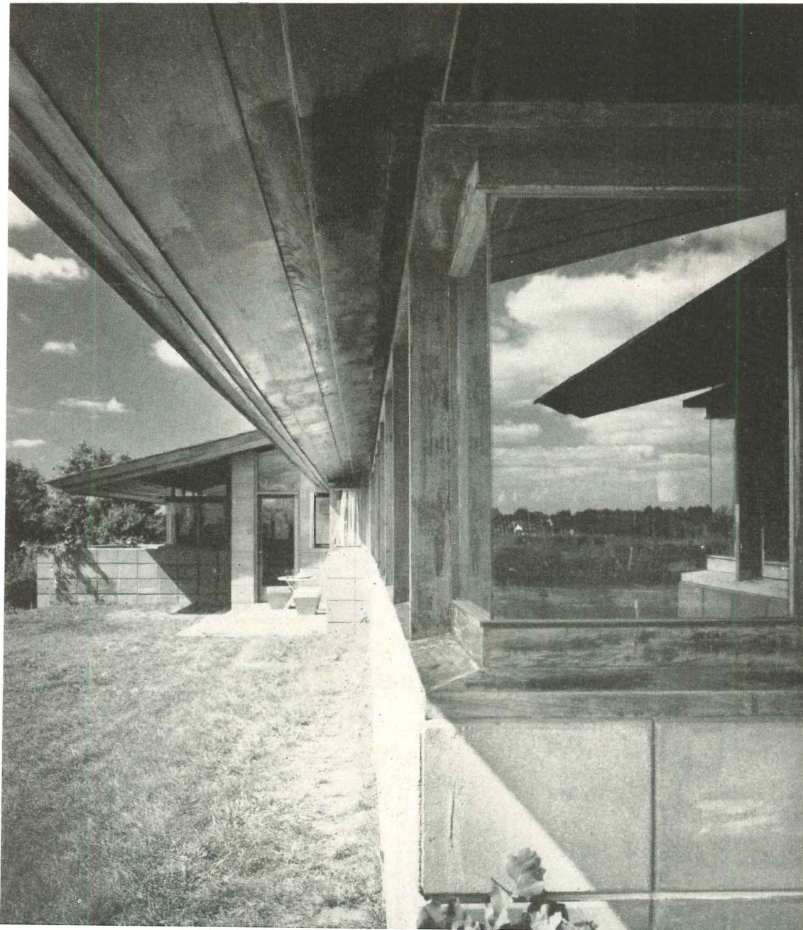
LIVING ROOM has ceiling of wide boards and battens that slopes out over windows to shield interior from sun glare. Glass door strip, left, keeps dining light and open. Room is U-shaped, (left), living and dining spaces wrap around masonry mass of central kitchen and dining area. Exposed floor slab is sealed and waxed.
