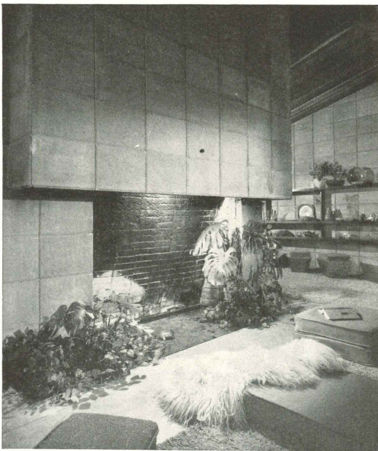
WINTER-SUMMER fireplace has the familiar broad lines and suspended masonry hood, plus a new wrinkle: hearth is sunk 6", has a drain and faucet which trickles water down on plants and fish pond during summer months.
