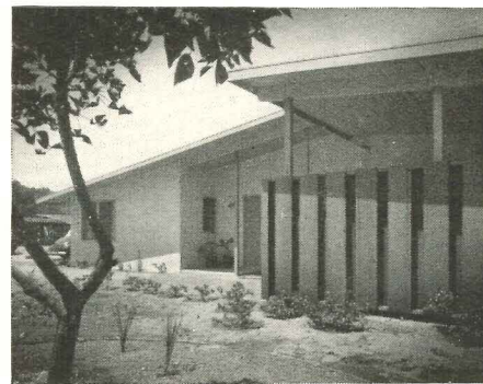
Post-and-beam construction of interior is reflected in porch and carport. House colors by William Manker are earthy browns, greens and yellows on exteriors and interiors.
