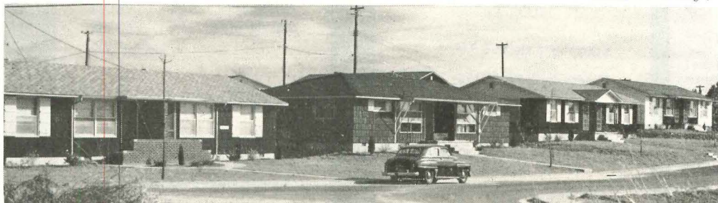
PRIZEWINNING EMPTY HOUSING: An NAHB Award of Merit went to Bralei Homes Inc. of North Little Rock for this defense housing project of 82 duplex units at Benton, Ark. Two bedroom apartments (750 sq. ft.) rent for $55 a month, $5 under the HHFA-imposed ceiling. At the end of January, 32 units were vacant—about the same rate suffered by two other projects nearby.
