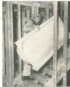
Made in white and pastels, the plastic tub is dressed off with a matching flat panel and a chromed metal strip.
