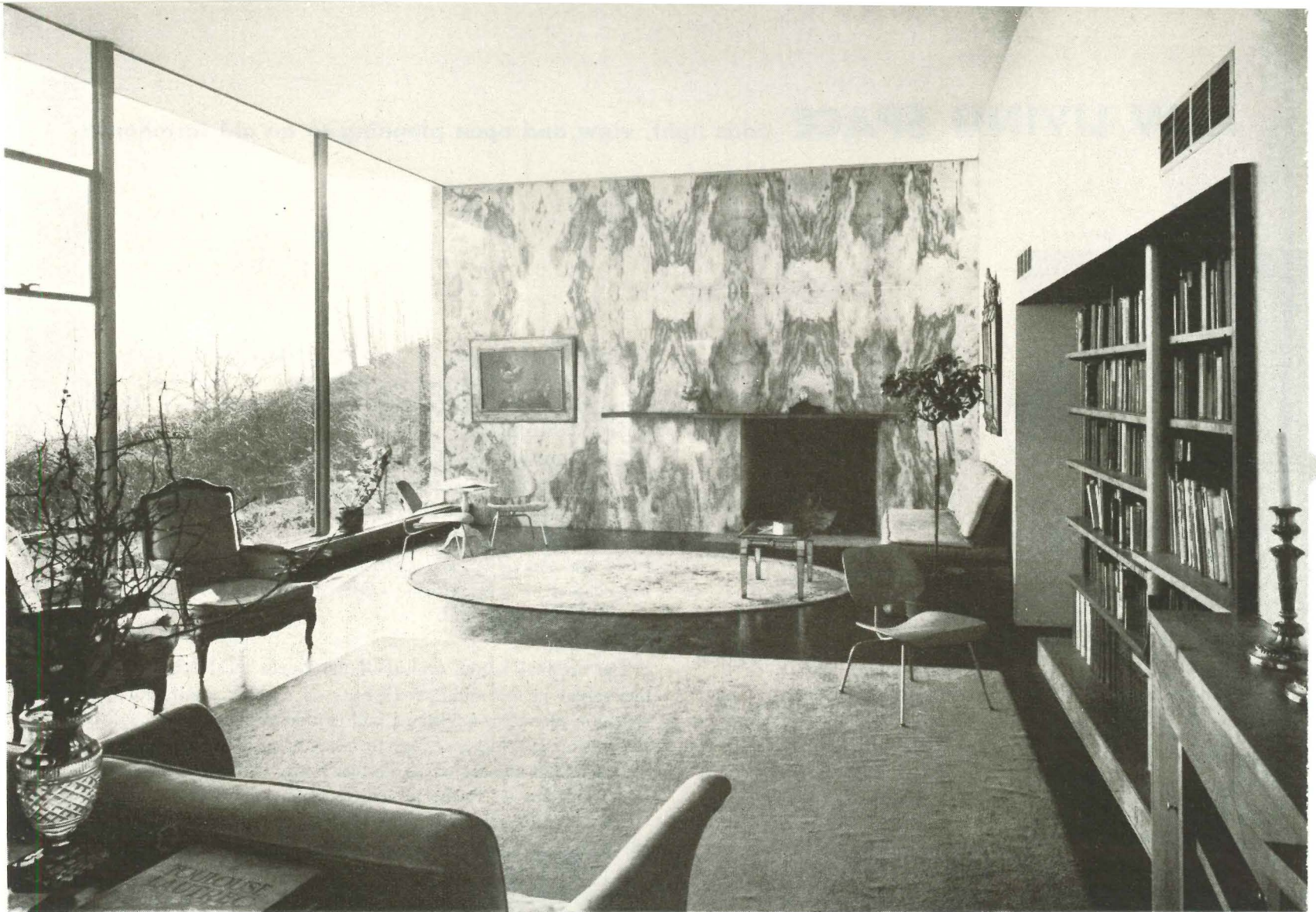
Polished formality is the mood in the big living room: dark walnut floor, walls of plate glass, pink-tan marble and white plaster. Large opening at right, with pipe column, is filled with bookshelves and door to playroom. Heating combines radiant baseboard pipes and warm air registers.
