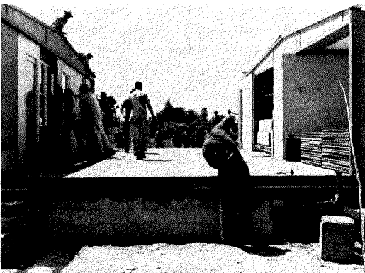
GRESHAM CONSTRUCTION CO. AND KNOX CORP. OFFERED CARL BERGSTROM HOUSE THAT EXPANDS ON SITE BY PULLING APART GABLE ENDS
