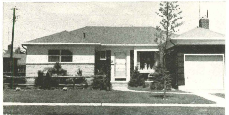
Sills and heads that don't line up make for incoherent facades
