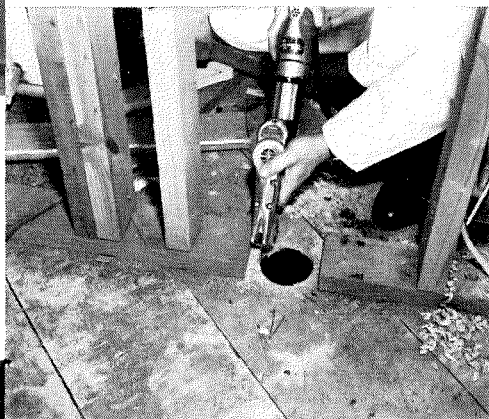
Less cutting is required for the passage of small pipes through floors. Framing construction isn't materially weakened. Builders report large savings in time and labor required to cut holes.
