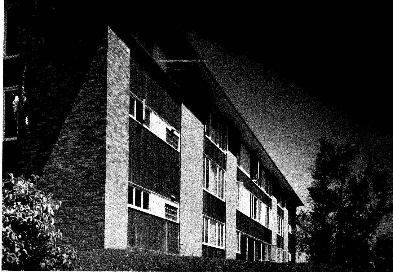
Brick veneer panels emphasize orderly window groupings. Spandrels are redwood siding. Slope beyond the lawn was left in a natural state.
