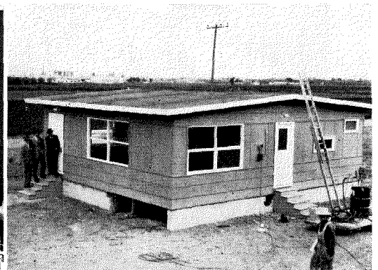
GRESHAM CONSTRUCTION CO. AND KNOX CORP. OFFERED CARL BERGSTROM HOUSE THAT EXPANDS ON SITE BY PULLING APART GABLE ENDS
