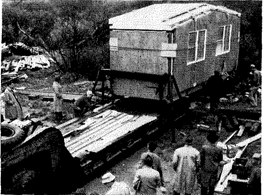
ACORN HOUSES OFFERED PORTABLE FOLDING HOUSE DESIGNED BY ARCHITECT KARL KOCH, TRANSPORTED AS AN 8' X 24' UNIT
