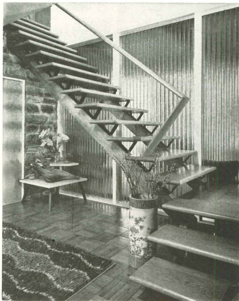
The stairs rise alongside a translucent glass screen and over the chimney wall to the floor above. Oak treads rest on triangular metal brackets screwed to 4" x 6" stringers. Oak parquet squares set in mastic make a "floating floor" over the radiant-heated ground slab.
