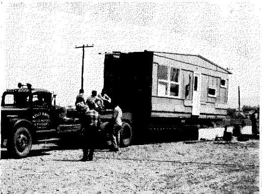
GRESHAM CONSTRUCTION CO. AND KNOX CORP. OFFERED CARL BERGSTROM HOUSE THAT EXPANDS ON SITE BY PULLING APART GABLE ENDS
