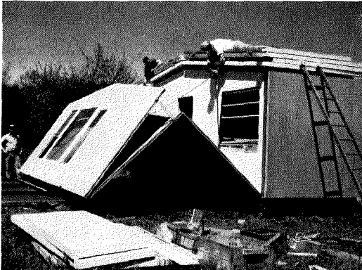
ACORN HOUSES OFFERED PORTABLE FOLDING HOUSE DESIGNED BY ARCHITECT KARL KOCH, TRANSPORTED AS AN 8' X 24' UNIT
