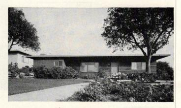
Flat-roofed version of the same house is finished with horizontal redwood and stucco. At the rear (below) big windows and sliding glass doors open the living-dining area to the paved terrace. Note depth of projecting eave which acts as sun shield.
