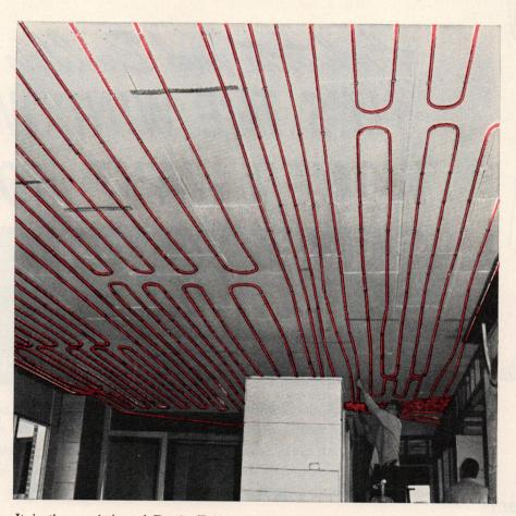
It is the conviction of Bundy Tubing Company that radiant heating grids rightly belong in ceilings. Among other advantages, *ceiling* installations provide proper floor warmth without danger of discomfort, respond far more quickly to thermostat demand, give a far *higher* percentage of radiant heat.
