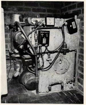
One of the great Levitt contributions to housing technology, this ingenious mechanism is the entire heating plant. Each year the Levitts have urged Engineer Jalonack to get the heater smaller. Working with producers York-Shipley, Jalonack achieved this model in 1952. Furnace, next to brick wall in kitchen, is size of washing machine, left, 30" high, 25" deep. A stainless steel top can be used as hot plate.
