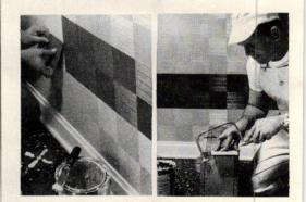
square is dabbed with mastic and pressed into place so none of the binder oozes through the seams. (Not a waterproof system, it is not recommended for use in baths or kitchens.) Retail price, not installed, is about  $60\phi$  per sq. ft. The finished wall may be washed clean, dusted with a brush or vacuumed. Colors, which go beyond the familiar pastels to include a deep blue green and coral, are permanent, and the material is said not to chip, peel, or crack.
