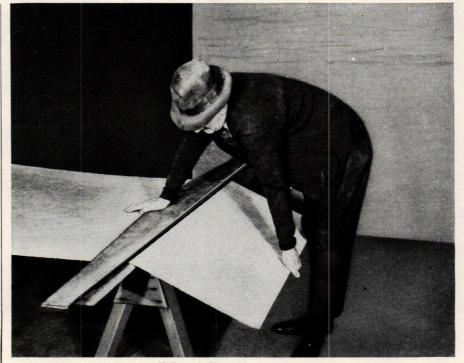
No need to saw Stonewall Board. Try this faster way. Just score it and snap it off. It breaks clean. Takes nails and screws readily. This method is not only easy to use, but time-saving and economical, too.
