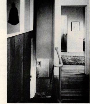
Gallery-effect stair landing was made by removing old bearing partition and replacing it with posts and parapet wall.
