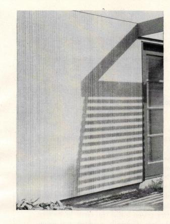
No feature of the new houses interests other builders more than the  $\frac{1}{3}$ " sheets of asbestos cement that form exteriors. Eight feet high x 32" wide, they butt together with an almost invisible crack. Produced in seven colors, vertical lines seem to be striations. At gable ends, top panels lap over bottom panels. Prepunched nail holes speed installation, let carpenters nail through into studs.
