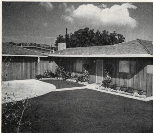
Most popular house has an L-shaped plan. The 12' x 14' study off the living room, thanks to its private bathroom and folding partition, is readily convertible into a third bedroom or guest room. Facade of this model is finished in vertical redwood boards which are also used for the fence and the screen which ties the house and garage together. Other walls are stuccoed. All house prices begin at about \$14,000, range up to \$17,500 depending on location and lot size.
