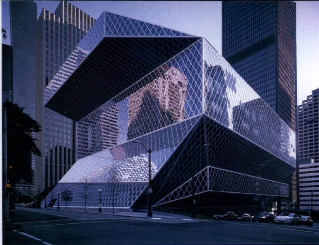
The oddly angled exterior of the Seattle Central Library, left, asserts itself within a canyon of banal office towers. ■ The diamond-shaped panes, below, are framed by diagonal steel grid work to brace the building against seismic shocks. ■ The stacks, below, left, housed in a continuous sequence called the books spiral, are brightened by overhead panels of light-diffusing plastic.
