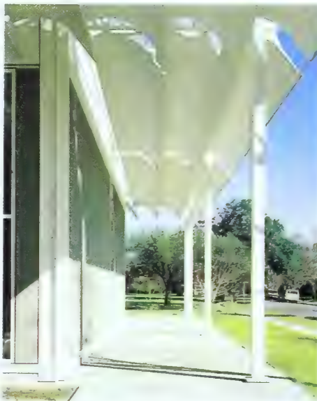
Top: The Menil museum is clad in gray-stained cypress and framed in white-painted steel. Above: Colonnade surrounding museum on all four sides is shaded by fixed ferroconcrete louvers.
