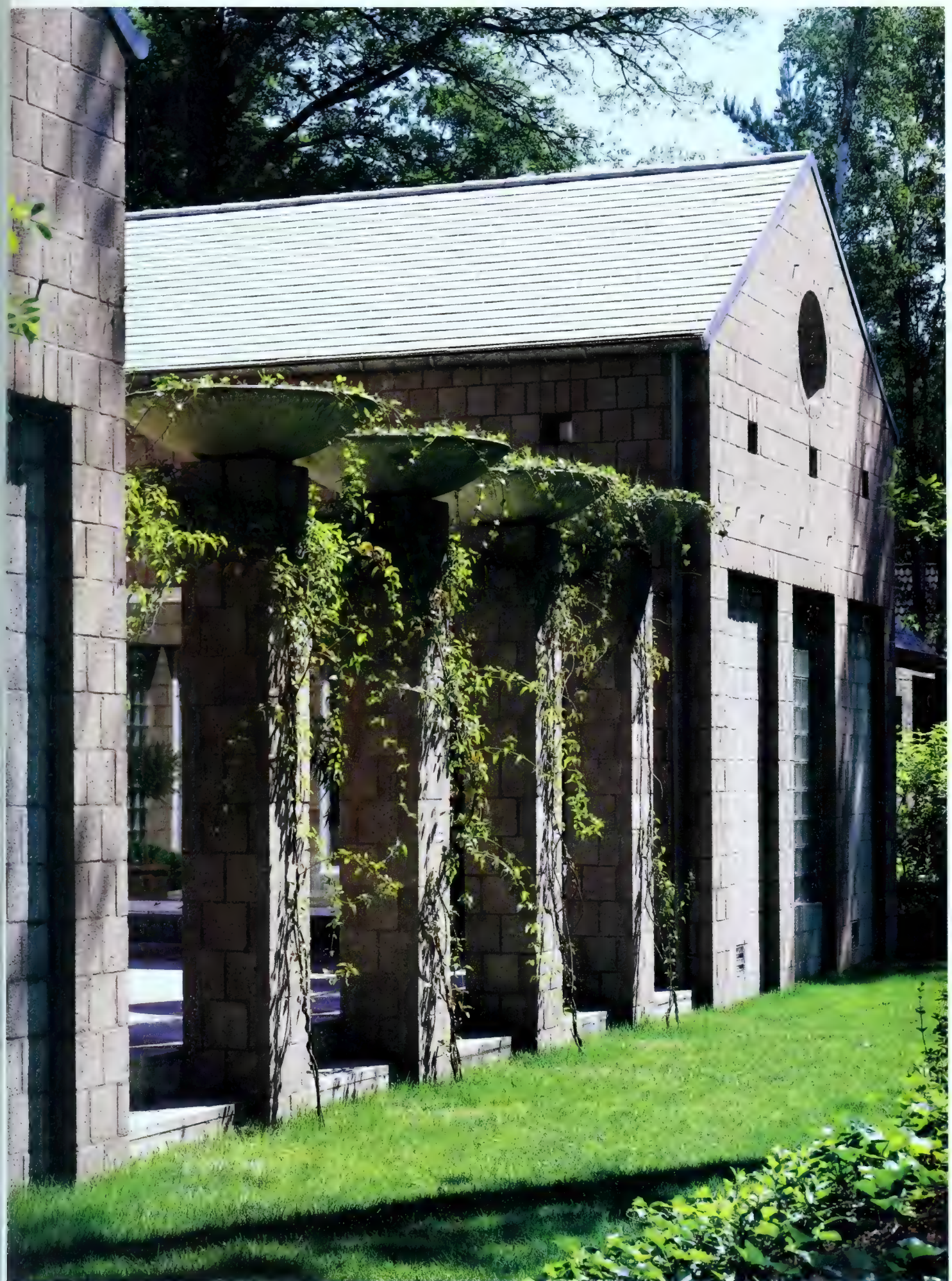
Pinkish blockwork, accented by gray, and four sentinel columns on the southern façade
