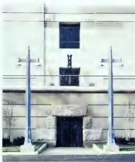
The limestone cladding of the new West Wing of the Virginia Museum is worked in a rich variety of contrasting textures.
