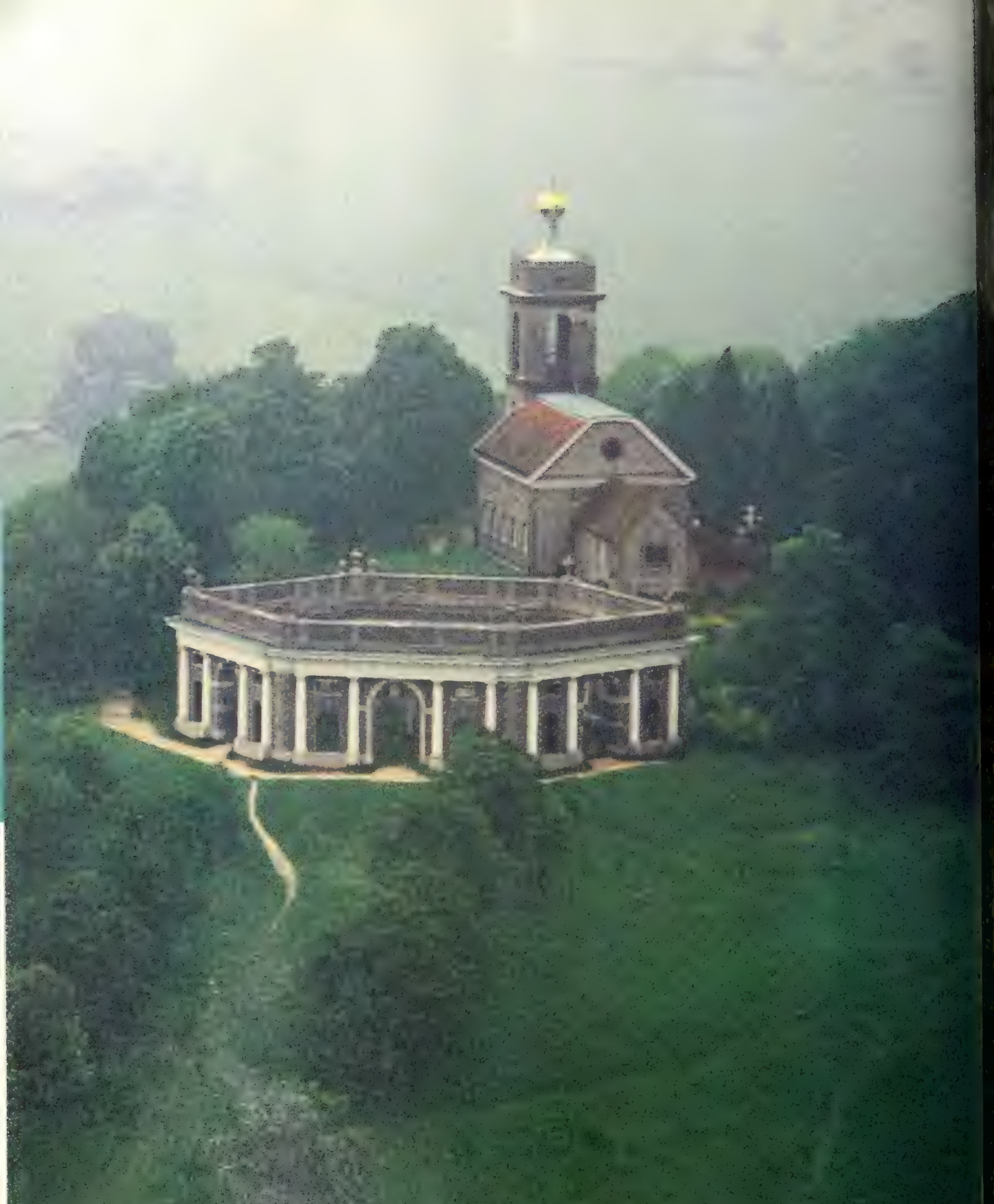
The Dashwood mausoleum and 13th-century church with tower rebuilt in 1751, inspired by Palladio's Customs House in Venice, the nave in 1763 after the Temple of the Sun at Palmyra. Opposite: Tapestries made by Josse de Vos, circa 1710, are reflected in a mirror in this State Dressing Room made for George III; a bit of ceiling made by Hannan based on those in Vatican loggia is also visible.
