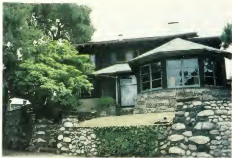
Brick and boulder retaining walls: a Greene trademark
