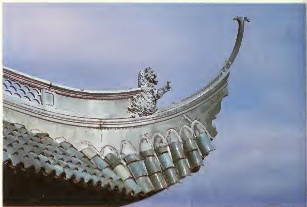
Plaster Foo Dogs decorate the tiled eaves of the teahouse—some are originals, others carefully made from recently cast molds.
