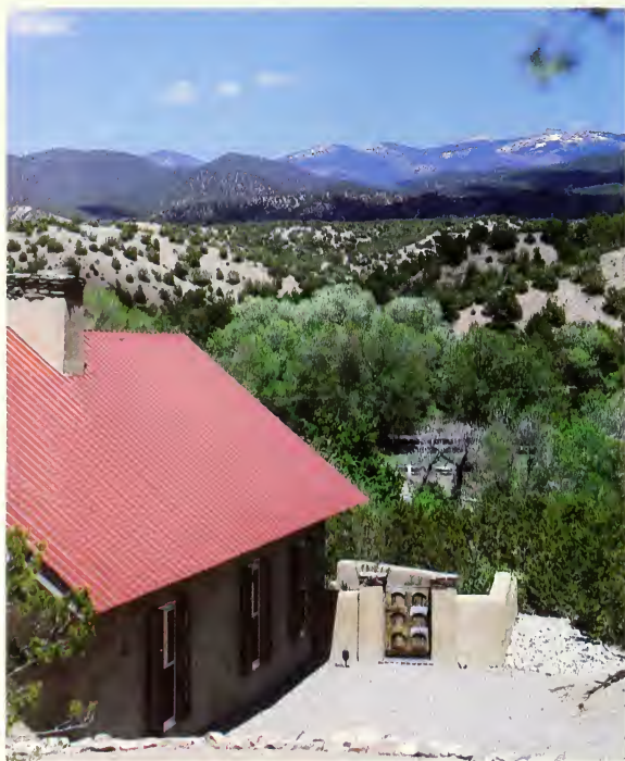
Above: A pitched roof covered by long-lasting tin—one of three over Betty Stewart's house—represents a stylistic revival that she has spearheaded in New Mexico, where most adobes have flat roofs. Chimney tops and gateposts are crowned by flat stones laid without mortar. Opposite: Carved birds appear in every room. This one by a fine Spanish-style pine bench in the entrance hall is a Canadian Indian example. Others in the collection are local, old and new; some come from New England.
