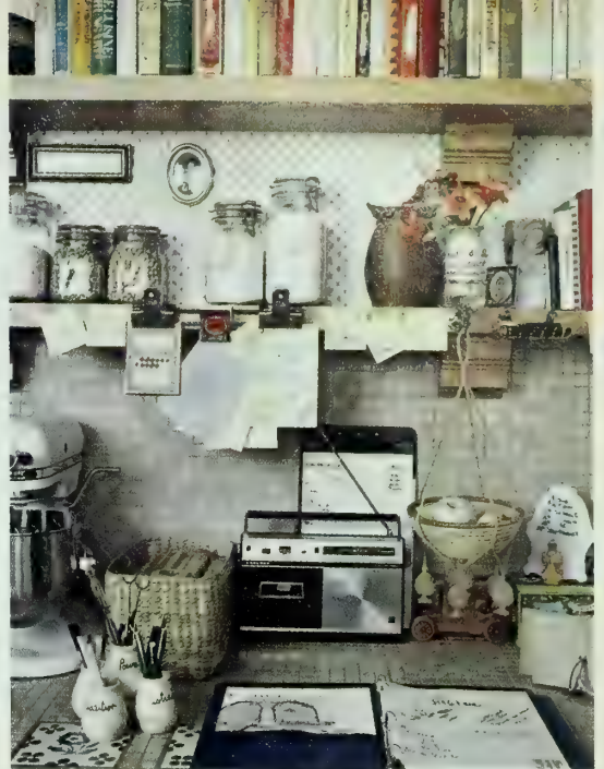
Shelves are two pieces of oak-veneer plywood glued together and edge-banded with 3/8-inch oak.
