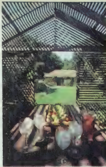
Left: The added-on slat house, designed by architect Peter Hoppner, provides shade for both plants and dining. Topped with plexiglass, it is useful even on rainy days. Workmen put in the foundation and roof; the Closes did the brick floor and framing. Facing it is Chuck Close's studio, with a roofline trellis for wisteria.
