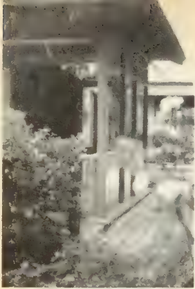
Approach to Mazzanti house
