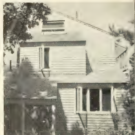
Prevailing breezes shaped the design of this tiny Martha's Vineyard house. Openings near the ground include windows, jalousie panels in the greenhouse, a screened porch, and adjustable wood flaps on the sheltered entry side. Almost all can be kept open in the rain.
