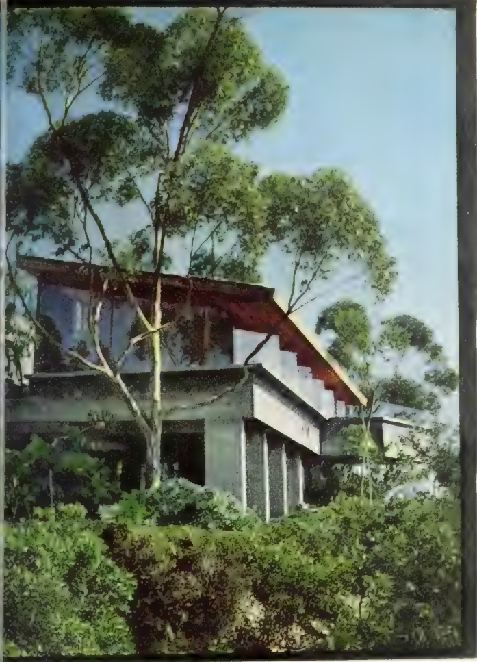
Upper story with zigzag glass panels along long wall as windbreak and for ventilation. Roof overhang shades room. Other half of house, at left, is studio wing; windowless wall encloses it on south.
