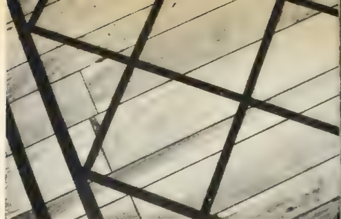
The finished floor, polyurethane-protected
