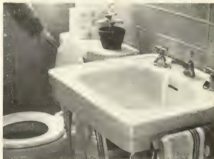
Turn on faucets, toilet to check water flow
