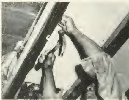
6. Rock lathe nailed between beams
