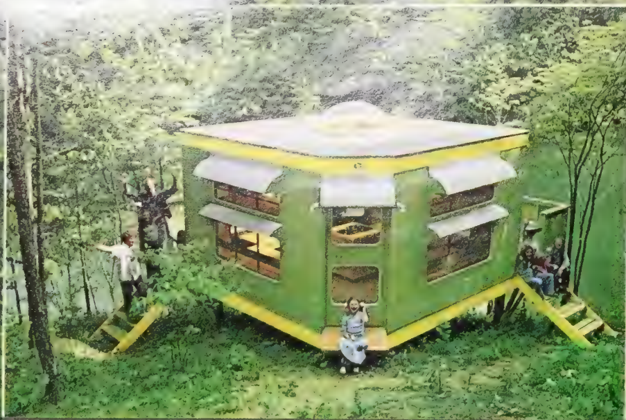
Awnings keep out rain; roof reflects sun. For light, screens, two doors, a bubble ceiling
