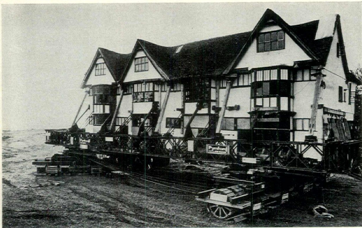
Above and left Pictures of Ballingdon Hall, Sudbury, Suffolk, en route from its 400-year-old site to new foundations, now being built, over half-a-mile away. See: THE HALL GOES SLOWLY UP THE HILL
