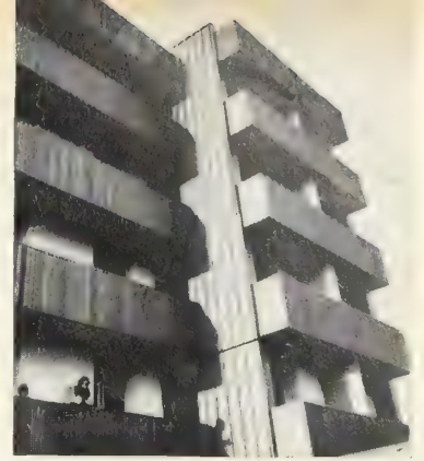
High-rise made of a stack of Stirling-Homex modules grows from the bottom: Whole building hydraulically lifted, new modules inserted beneath.
