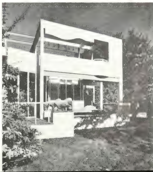
Adding new wing spurred remodeling in existing downstairs. Walls between rooms were replaced by steel posts and beams; kitchen was rebuilt around center cooking island.
