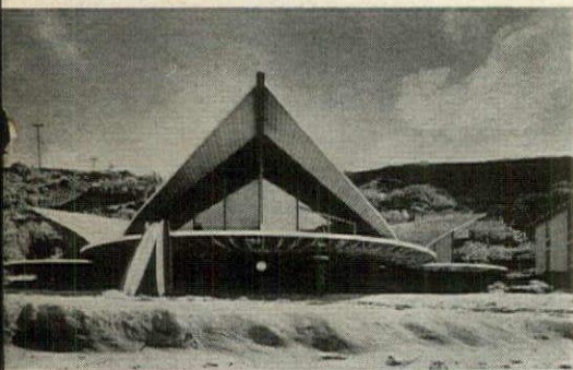
Central arched area, 18 feet high at its apex, is the living room. In the smaller, adjoining areas are the music room at left, and at right, oriented to sunrise, the breakfast room.
