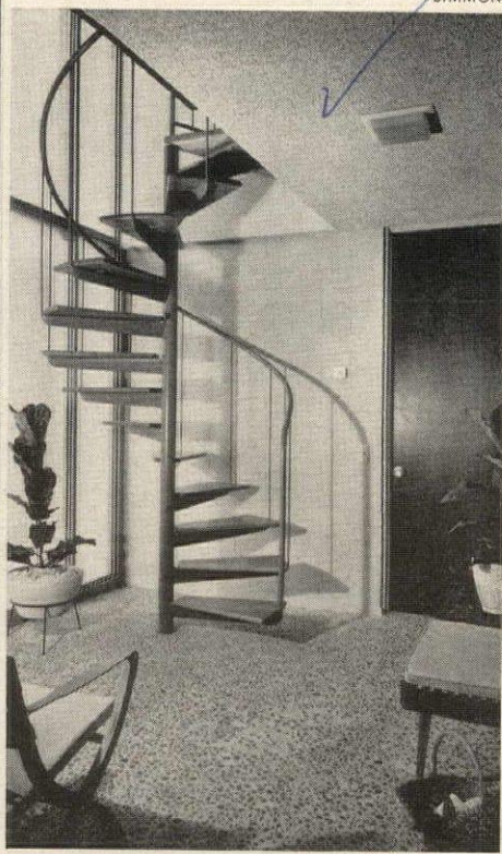
In the hall, a spiral steel staircase makes a graceful ascent to bedrooms. To muffle the boom of pounding surf, all ceilings are of sprayed acoustical plaster.
