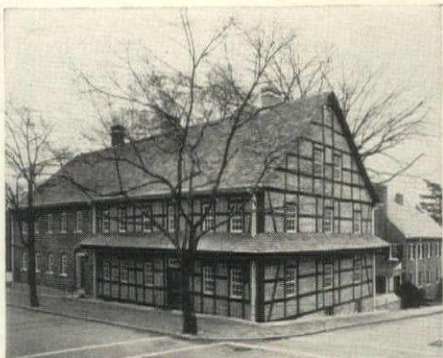
Earlier (1769) half-timbered portion of Single Brothers House is remarkable for a feat of workmanship: timbering was raised in only two days.
