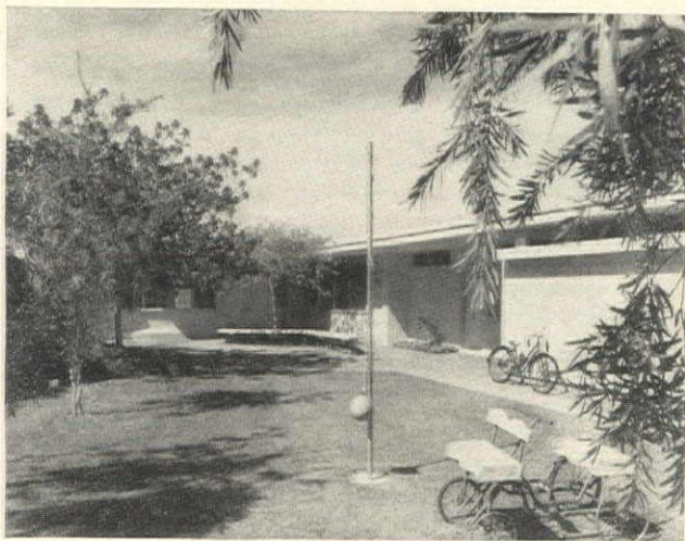
The children's play yard (which is separated from the entrance garden by their own rooms, and from the swimming pool terrace by the laundry and maid's room) has the only lawn about the house. At the right is a long storage wall for bicycles and garden equipment.
