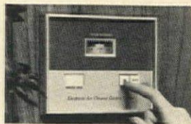
Living-area control panel
