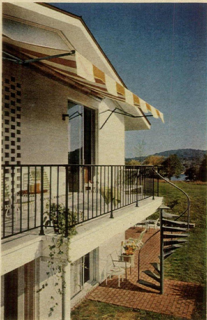
IDEA: a spiral staircase to link master bedroom balcony and terrace; a pierced brick wall to admit daylight, yet guard privacy of master bath See pages 103 and 114
