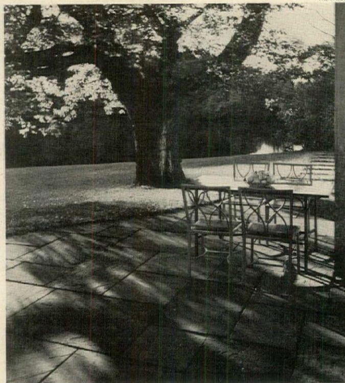
CUT SANDSTONE in modular pattern is most formal terrace material, offers a great variety of combinations with but three or four different sizes. May be laid dry (as here) or in mortar.
