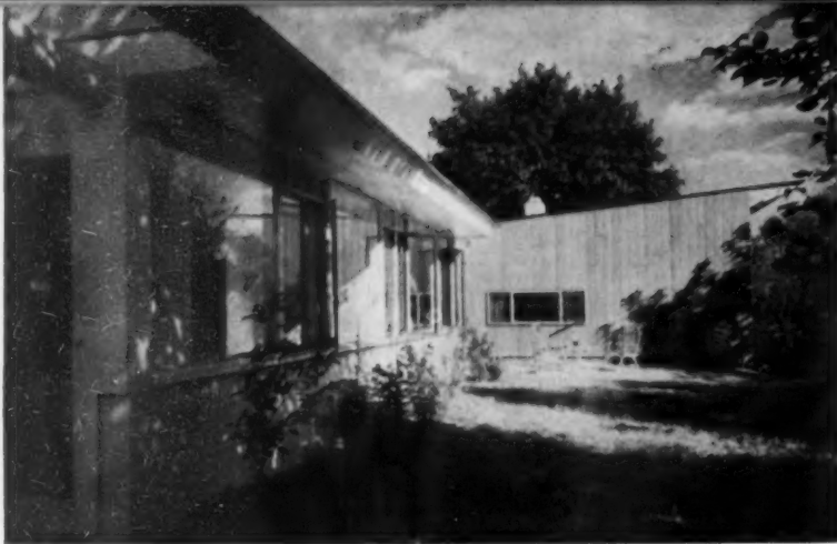
SOUTH TERRACE IS SHELTERED BY THE HOUSE
