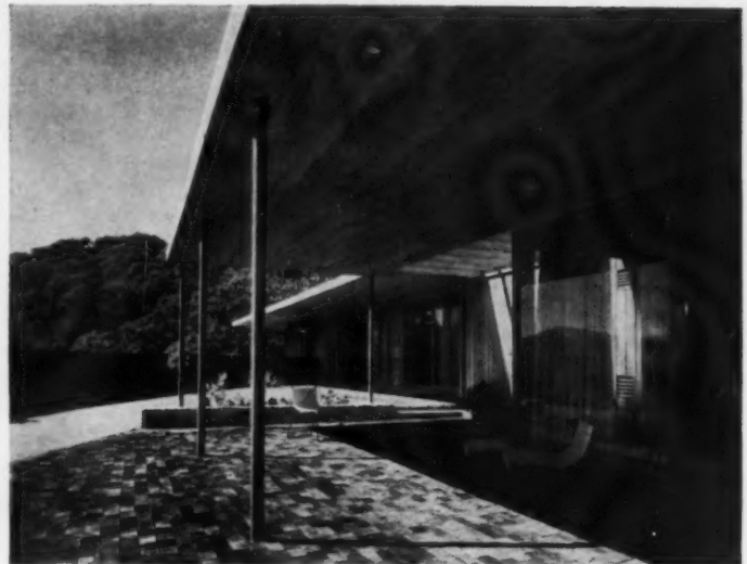
WIDE EAVES shelter the outdoor living room. The wood block paving is comfortable for barefooted swimmers: not too hot at midday, it retains the heat after sunset. The bedrooms are beyond the raised flower bed.
