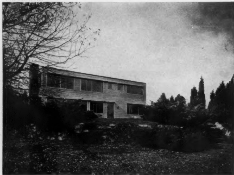
ON THE GARDEN SIDE the main rooms look out to a view of Narragansett Bay. Narrow projections over the windows keep rain from dripping on the glass.
