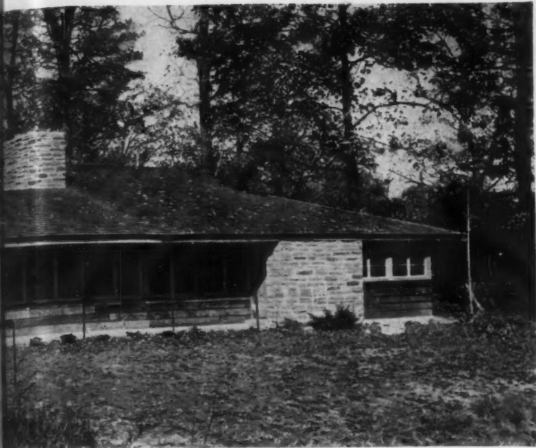
WIDE EAVES project beyond the southeast wall of the house, shading the entrance walk and protecting dining room, living room and study windows from the glare of direct sunlight. The roof extension, opposite, forms a covered porch and carport. Mineral wool insulation in roof and double glazing in windows cut the Turners' heating expenses during the winter months.
