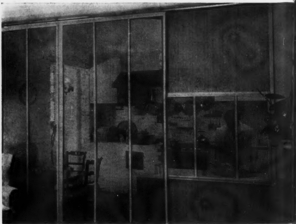
TWO SIDES OF THE SAME SCREEN. At the left , a cook's eye view through to the living room, with the central panels of the screen pushed open, along their overhead trolley. Serving counter top opens to twice the size shown. Above , guest's eye view of dinner preparation, with the cook, a shadowy, unobtrusive figure, glimpsed vaguely through the open mesh of the cane panel screens.
