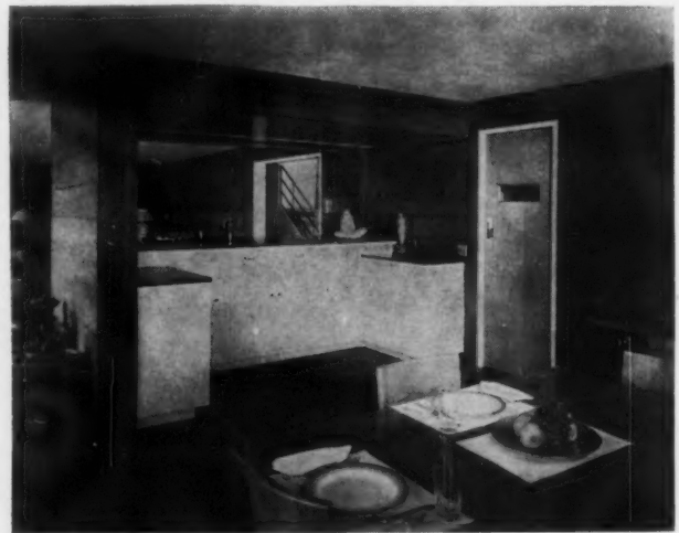
THE DINING ROOM is separated from the living room by a built-in bar and a cypress-slat blind which rolls up into a ceiling pocket in the manner of an old-fashioned roll-top desk.
