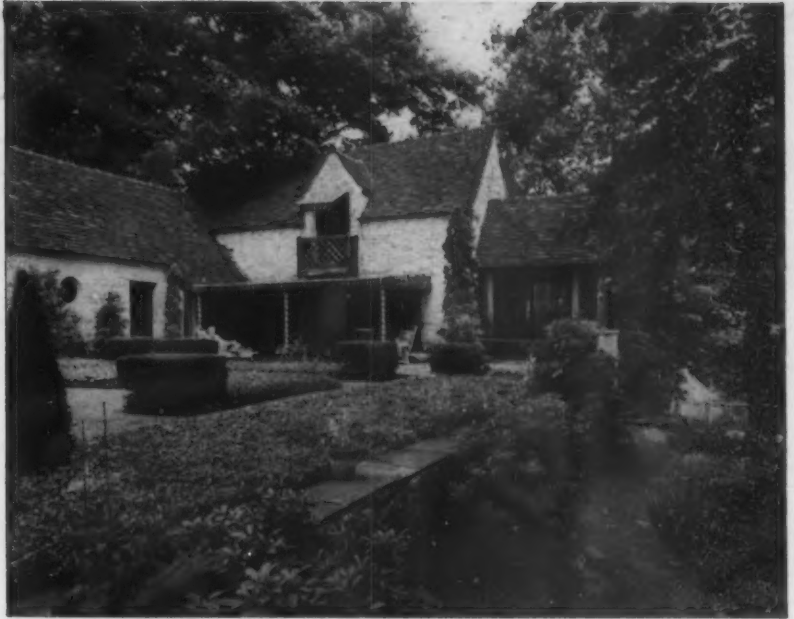
THE HOUSE is of hewn stone, has a hand-made tile roof
