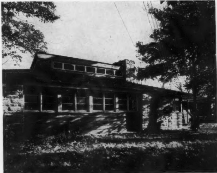
ROOF-LINE window band facing northwest augments daylight entering the living room and supplies center of the house with ventilation.
