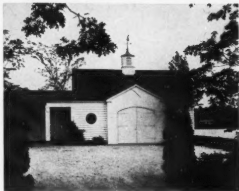
A COVERED PASSAGEWAY links the garage-boathouse and the library in the downstairs wing.
