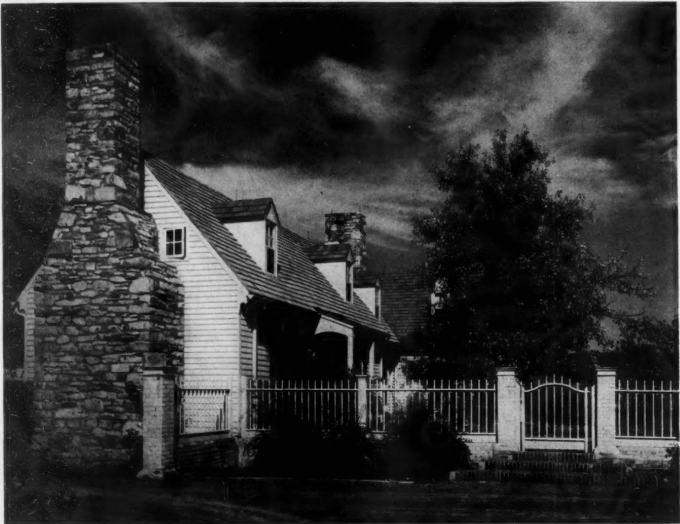
MAIN PART OF THE HOUSE was rebuilt from an early cottage. The sturdy chimney, steep pitched roof, clapboard walls duplicate old Williamsburg design. Entrance porch, fence and dormers are new but in the same character.
