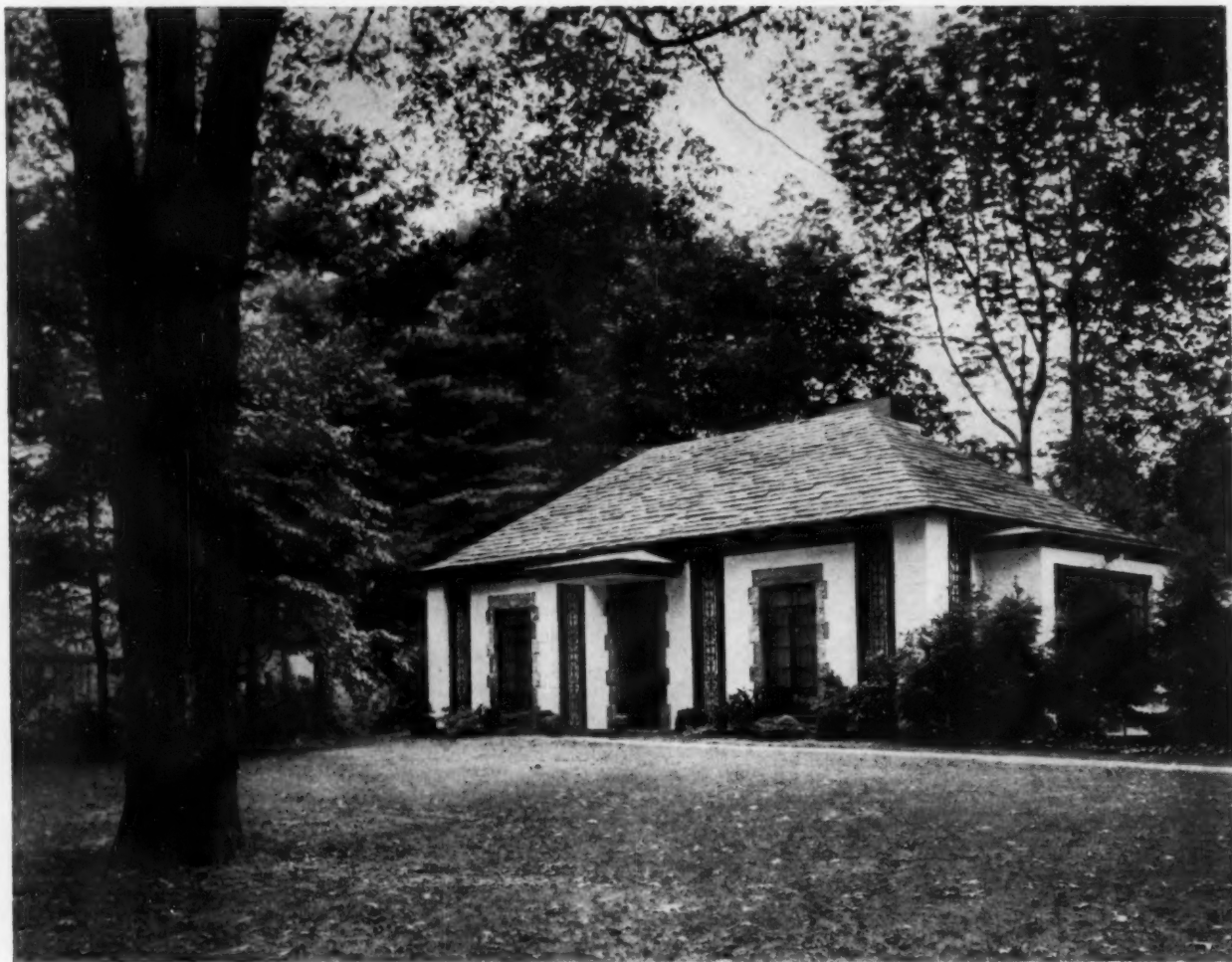
White painted brick alternates with wrought iron grillwork to enliven Mr. and Mrs. Dowdle's Connecticut house
