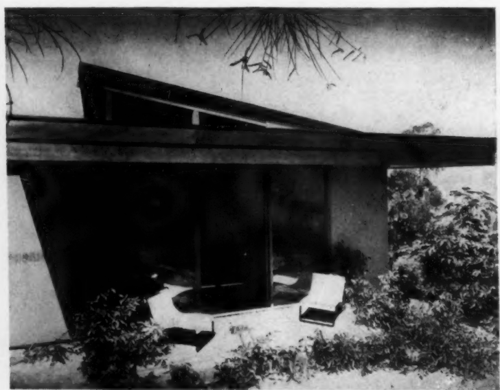
TERRACE OFF BEDROOM, perched on a ledge overlooking the city below, is shaded against full sun by wide roof overhang. One of the glass panels slides open on metal tracks. Small top windows open readily.
