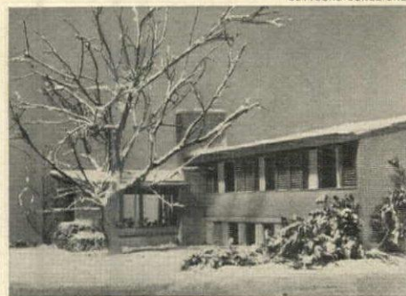
Essence of split-level planning is shown in this view of Mr. Yost's design which puts the living room half way between bedroom and basement floors. Shown at the TOP OF THE PAGE is the living room and porch view.
