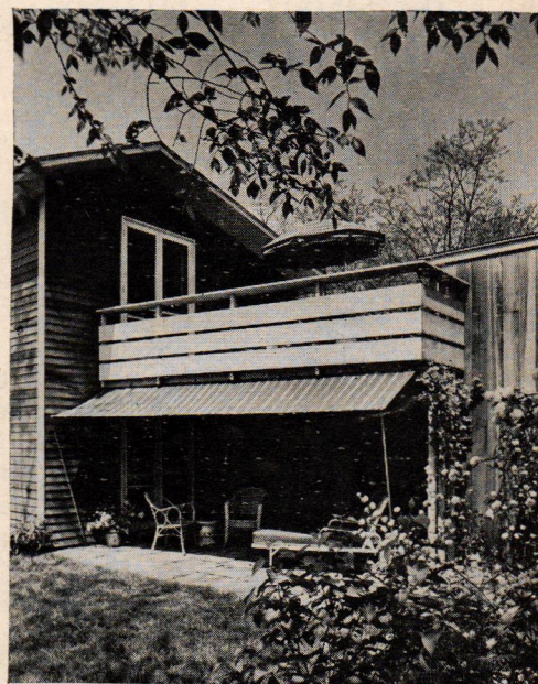
Detail of terrace and upper deck
