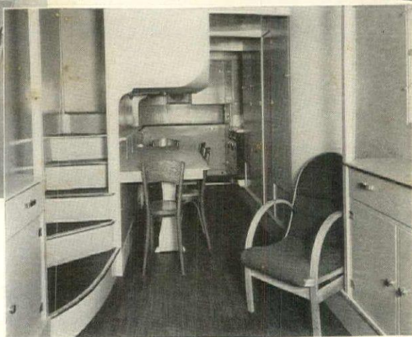
For low cost shelter midway between the trailer and a fixed house, Corwin Willson has designed this two-story portable structure. It is conveyed to the site on a wheeled dolly, then jacked up on six piers and connected to utility outlets. Upstairs ( far left ) are four beds and a bath. Downstairs ( left ) is a living-dining room, also equipment for heating, cooking and washing
