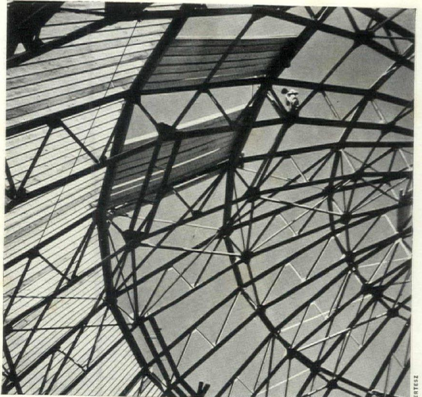
STRUCTURAL STEEL HAS LONG BEEN A PRIME FACTOR IN INDUSTRIAL DESIGN
