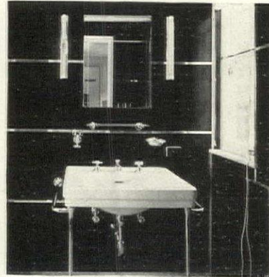
Large sheets of plywood or building board, plastic-faced, may provide an inexpensive shell for future rooms
