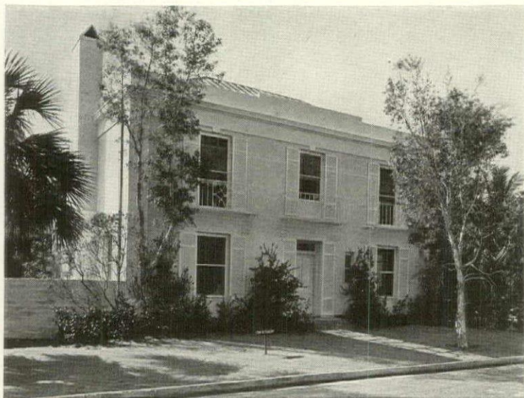
PENDLETON AVENUE HOUSE AT PALM BEACH
