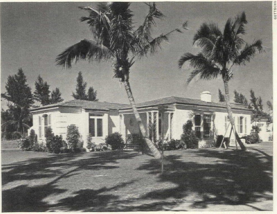
RESIDENCE OF H. BERMAN, MIAMI BEACH
