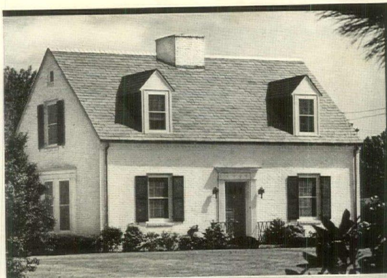
Cabot's DOUBLE-WHITE on brick on a charming little house at Manhasset, N. Y. (Blinds and trim painted with Cabot's Gloss Collopakes). Architect, Reinhard M. Bischoff, N. Y. C.
