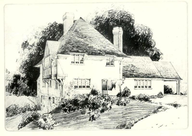
Of the English cottage type, this house is of cinder-concrete block construction covered with stucco surfacing. The roof is of rough slates laid in an irregular manner. The slope of the ground on one side of the house allows the garage to be in the basement
