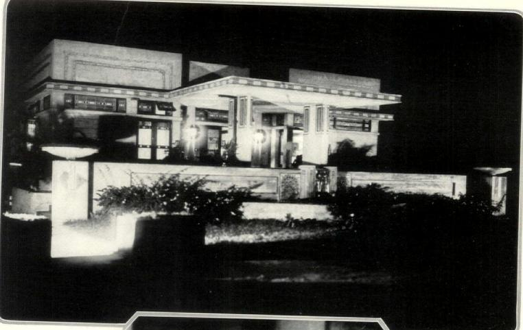
Both the inside and outside walls are concrete rubbed down. No plastering was used. The windows are casements filled with leaded glass. All floors are tiled. Outside lighting is designed so as to throw the mass of the house into sharp relief against the tropical night
