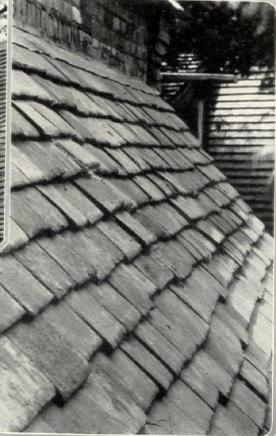
(Below) A close-up view of the roof showing the rough shingles and irregular lines produced. The shingles are of rough tile and in color range through various shades of reds and browns. They vary in size and thickness
