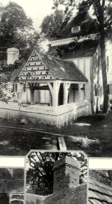
The texture obtained by the roof may be seen from this picture which was taken from a distance. This roof treatment was used to simulate the effect obtained from many years of weathering
