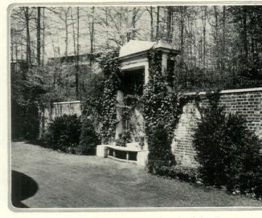
The severity of a garden wall is relieved by the very decorative niche shown above. The wall is of red brick and the niche of concrete and terra-cotta backed with brick
