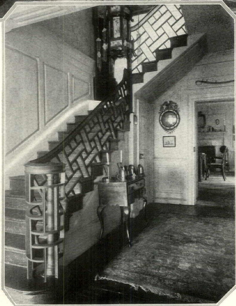
The principal feature of the entrance hallway is the mahogany stair-rail carved in an extraordinary design by John Bowen, a King's convict, who was also the artisan of the more conventional paneling and carving elsewhere in the house
