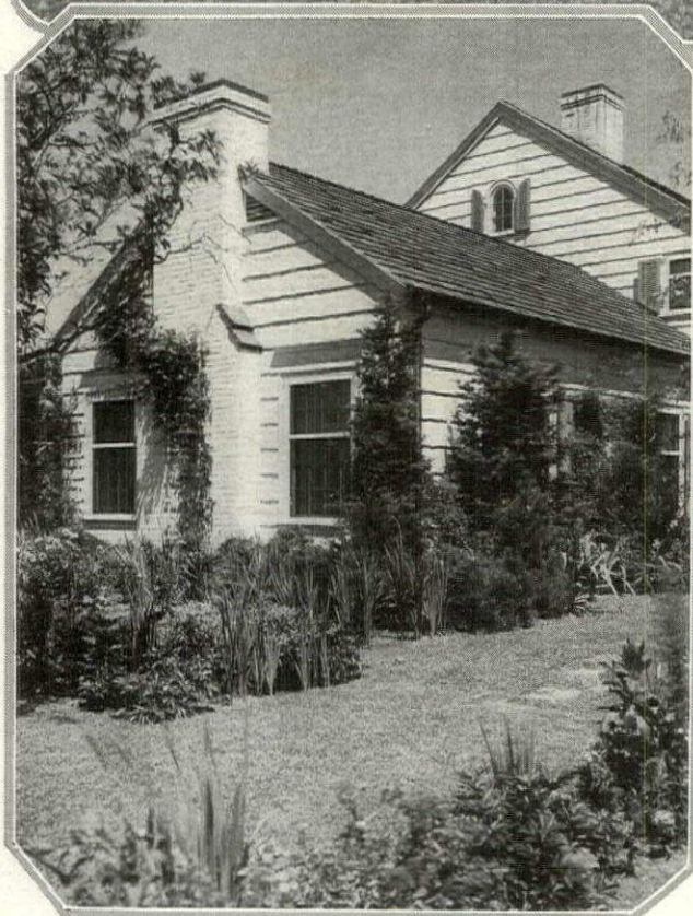
A detailed view of the living room wing shows the materials of the house and their treatment. The walls are shingled and stained white; the bricks of the chimneys are painted white and the solid paneled shutters are apple green. The ever-green planting of tall Conifers may soon be too robust
