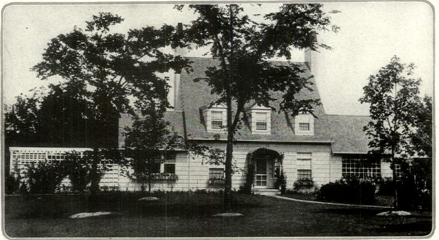
Above is shown the house after it had completed the first stage of its development from farmhouse to, ultimately, a country house of considerable size
