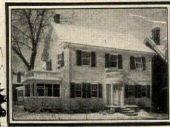
Exterior of Redwood Residence at Minneapolis, Minn. Everett Addy, Architect
