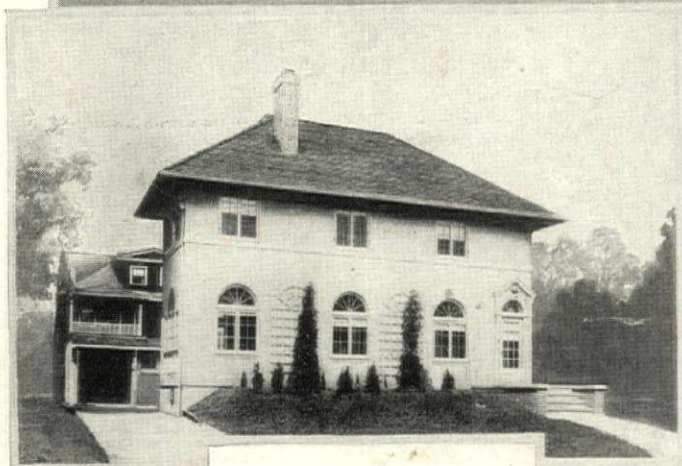
Owners, Architects & Builders, The Joseph Larong Co., Cleveland, O.
