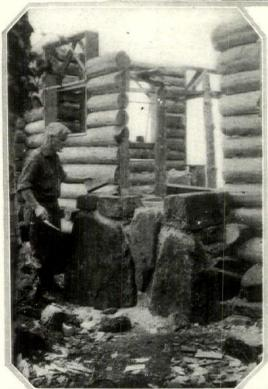
Here the project begins to take form. The layout of the floor logs reveals the shape and size of the cabin, and the method of framing
