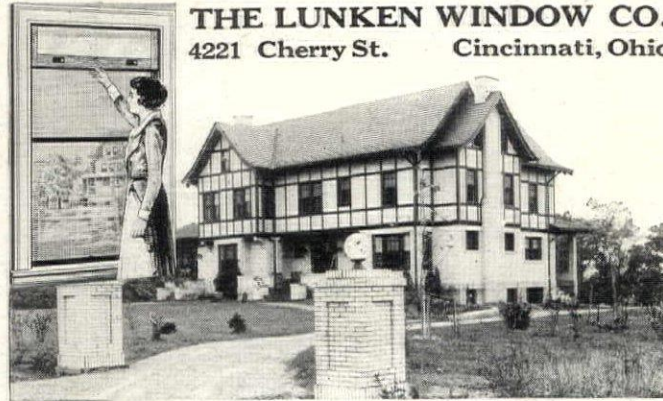
Lunken Windows Installed in Residence, Mr. Weise, Bridgeville, Pa.
