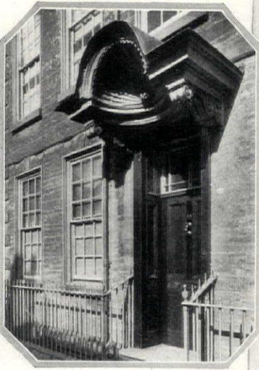
This shell-hooded doorway, with carved console brackets, in Buckinghamshire, England, is characteristic of the vigorous style of its 1680 period
