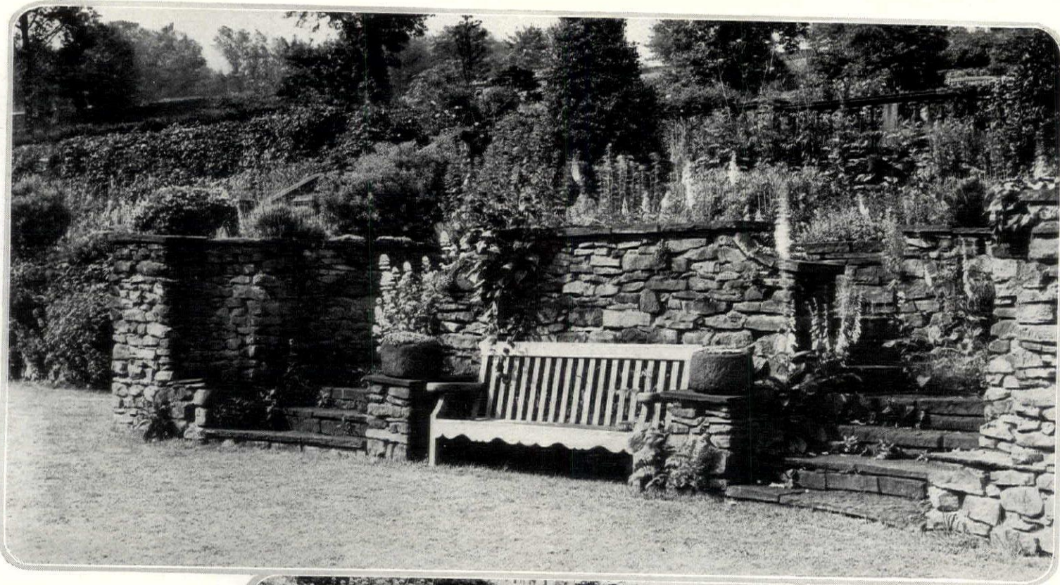
A double stairway, interestingly designed, and constructed of dry masonry in which wall plants are used, forms a splendid end to its garden
