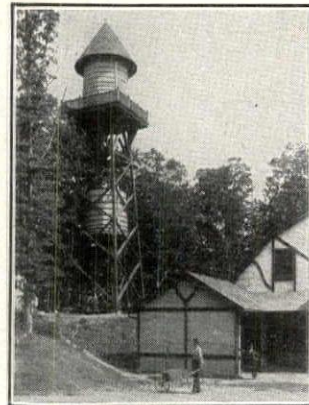
CORCORAN TANK TOWER
